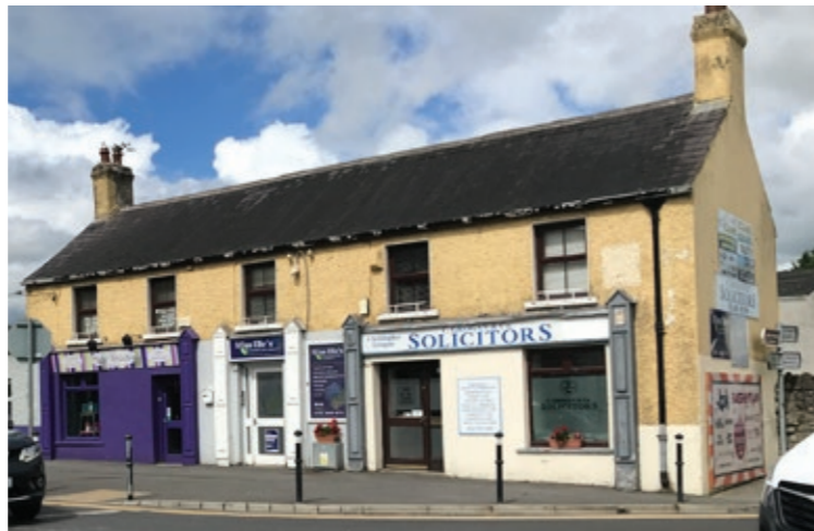
Examples of shopfronts for improvement
