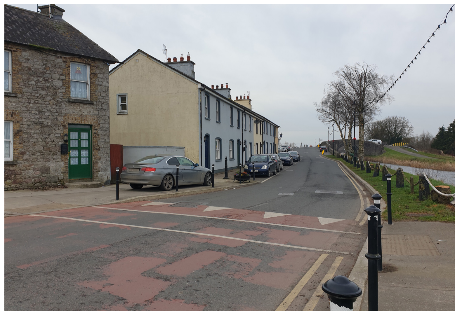
Road space and pedestrian realm with potential for improvement
