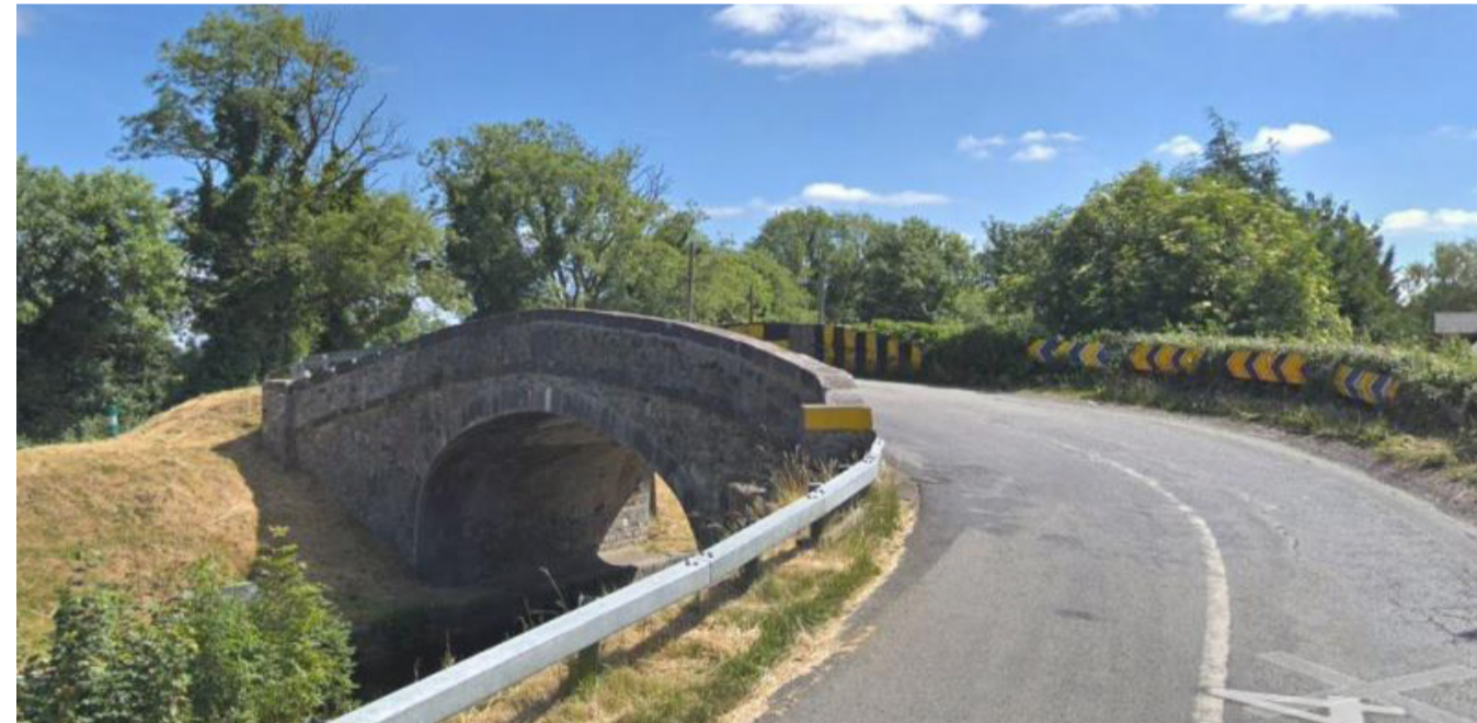
Skew (Shee) Bridge
