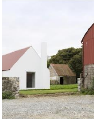
Contemporary use of corrugated sheet metal roofing (Image Ryan Kennihan Architects).
