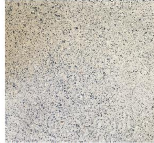
Ground concrete surface finish.
