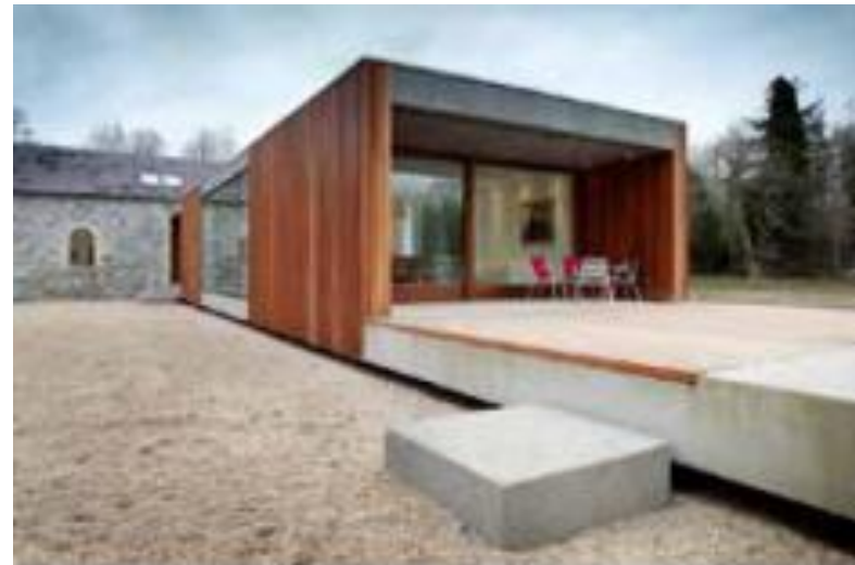
Figure 8.1 – Refurbishment and extension, Ballymahon House (ODOS Architects).
