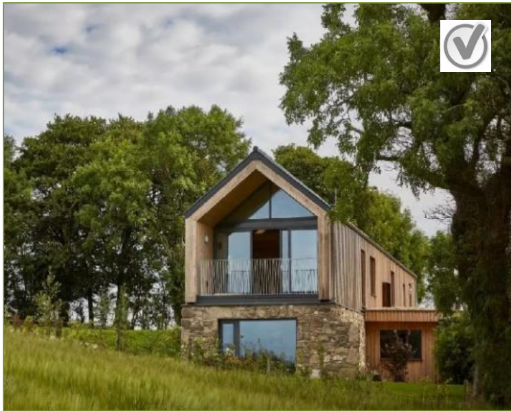
Figure 3.6: A narrow plan house design on a sloping site maximising existing screening.
