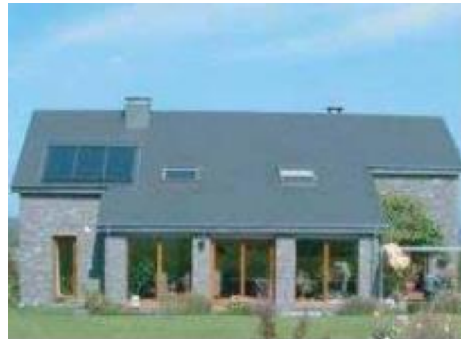
Figure 6.1 – Image of roof solar panel.
