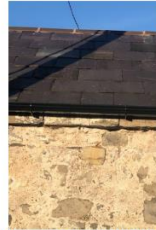
Natural slate, coursed rubble with lime render.
