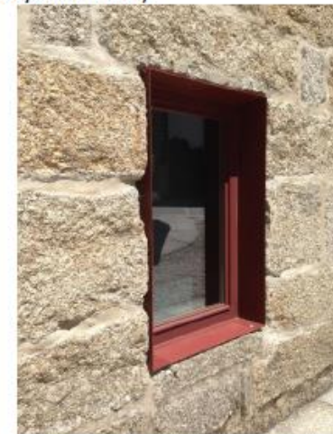
Contemporary window with painted steel reveal.
