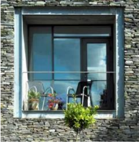
Figure 5.17 – Successful combination of traditional and contemporary materials. Castlegrey. Denise Murray, Murray O’Laoire Architects.
