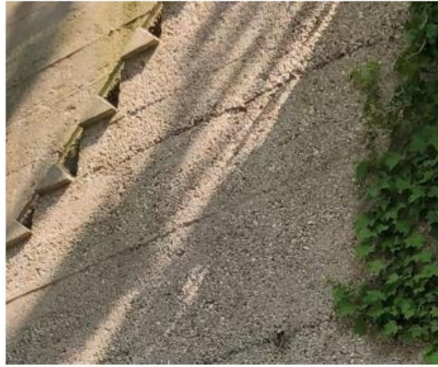
Rough cast concrete.
