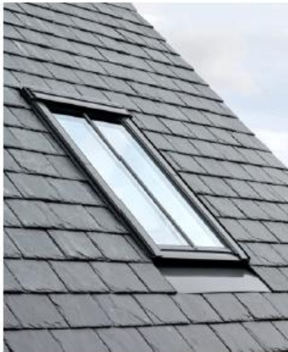
Flush 'conservation' rooflights..
