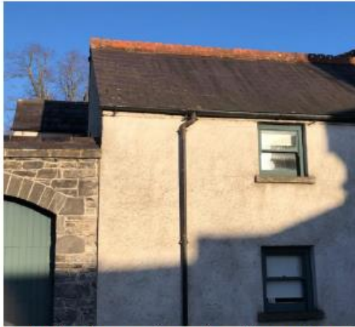
Natural slate, lime render and cast-iron rainwater goods.
