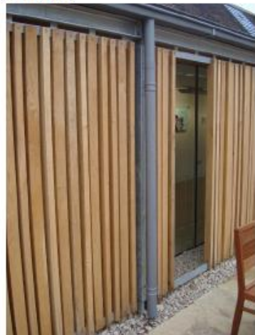
External timber – untreated larch.
