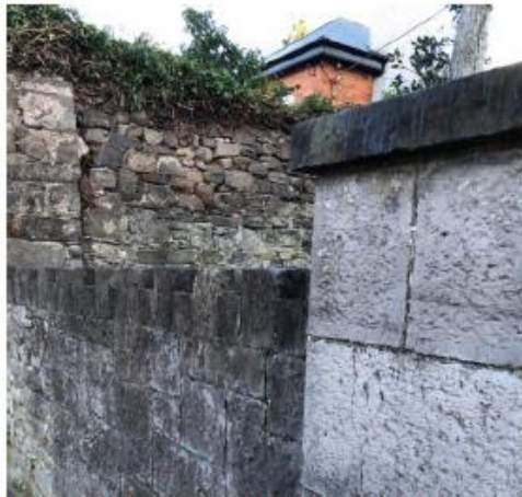
Random rubble, coursed rubble and ashlar stonework.
