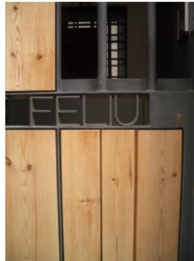
Contemporary steel and timber gates.
