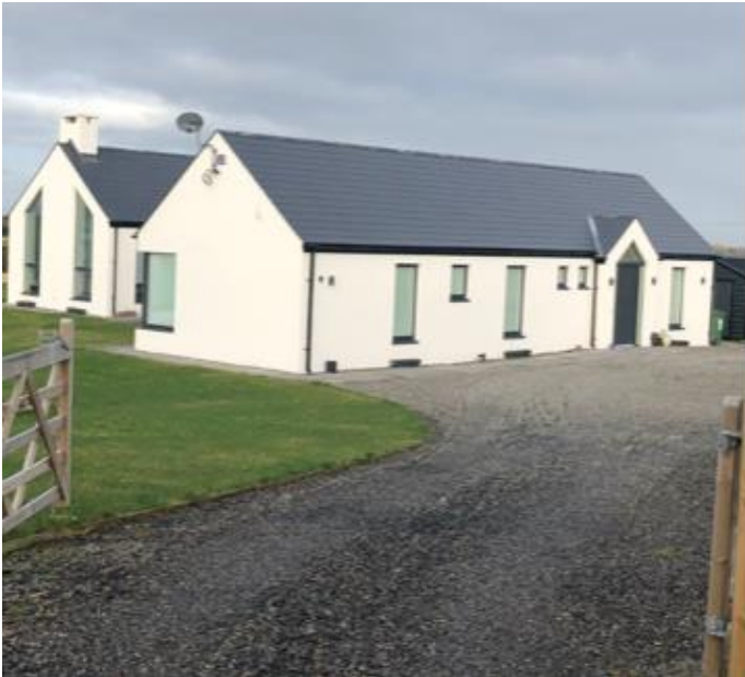
Figure 7.5 – Example of a driveway surfaced with permeable material (Straffan, Co. Kildare).
