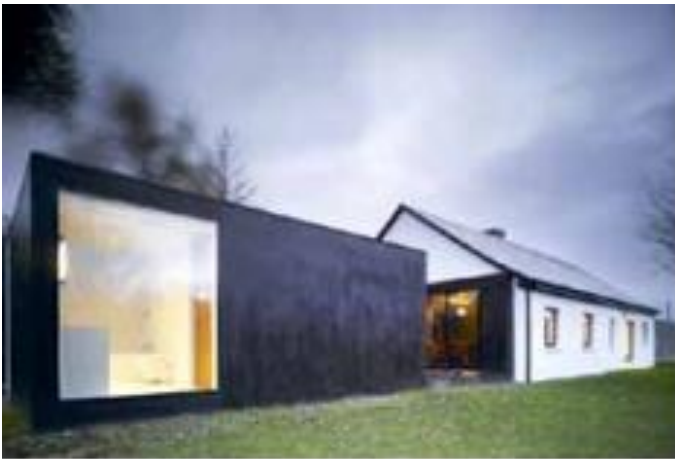
Figure 8.3 – Extension to side of house. Glengowla, Co. Galway (Boyer Kennihan Architects).
