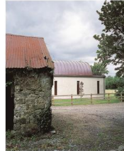
Standing seam copper roofing. (image: Aughey O'Flaherty Architects).
