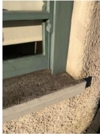
Painted timber, dressed limestone and lime render
