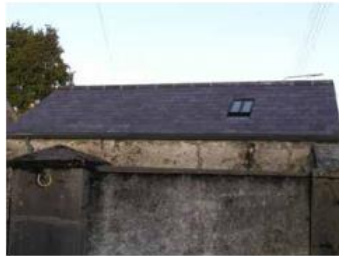
Figure 5.5 – Example of traditional rooflight flush with slate detail; Naas, Co. Kildare.
