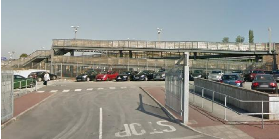
Figure 8.36 Existing Wheelchair Ramp Infrastructure at Sallins Station
