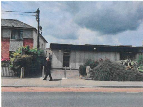
Fig 5: Existing extension and adjacent dwelling
