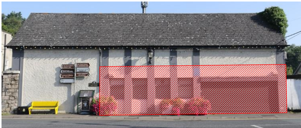
Plate 19: Front facade showing area where original walling has been removed
