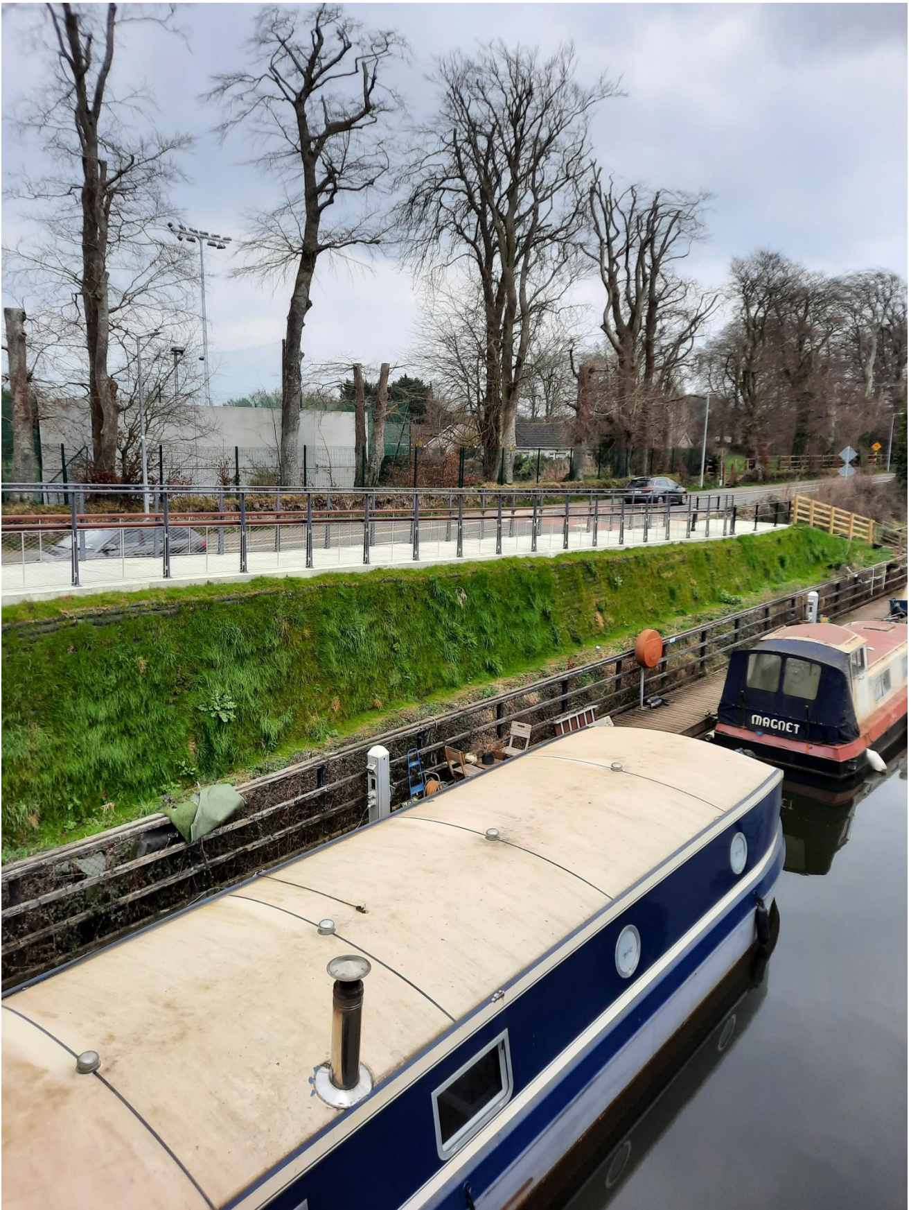
Figure 3-8: Green Faced Reinforced Earth Approach Ramps (Sallins)
