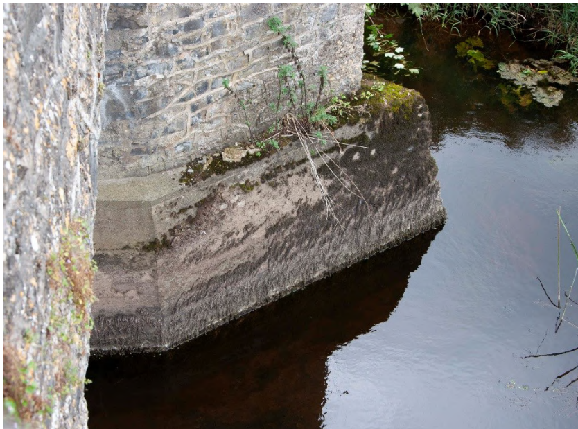
Plate 16: Close-up of concrete base of triangular cut-water/pier
