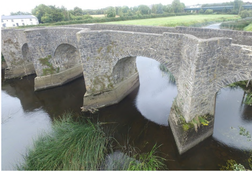
Plate 14: View of triangular cut-waters on north-facing elevation
