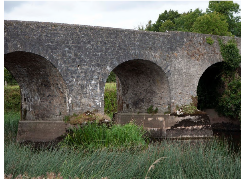
Plate 15: View of triangular cut-waters on south-facing elevation, with rendered soffits visible
