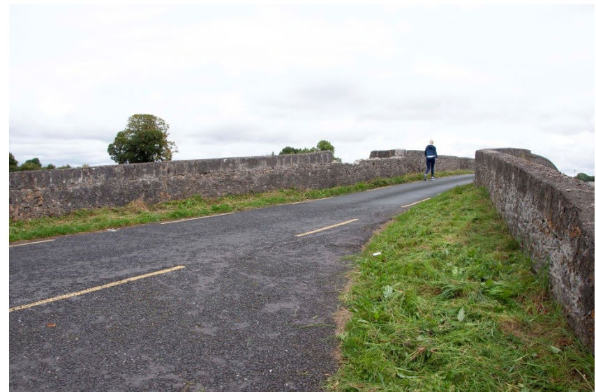
Plate 25: Approach walls on west side of bridge, looking northeast
