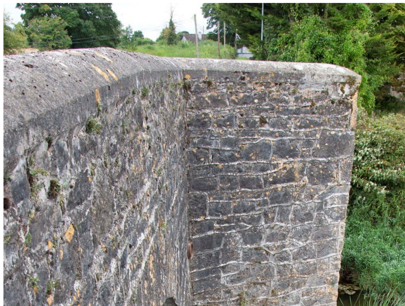
Plate 24: Detail of cut-stone coping on parapet wall and triangular cut-water
