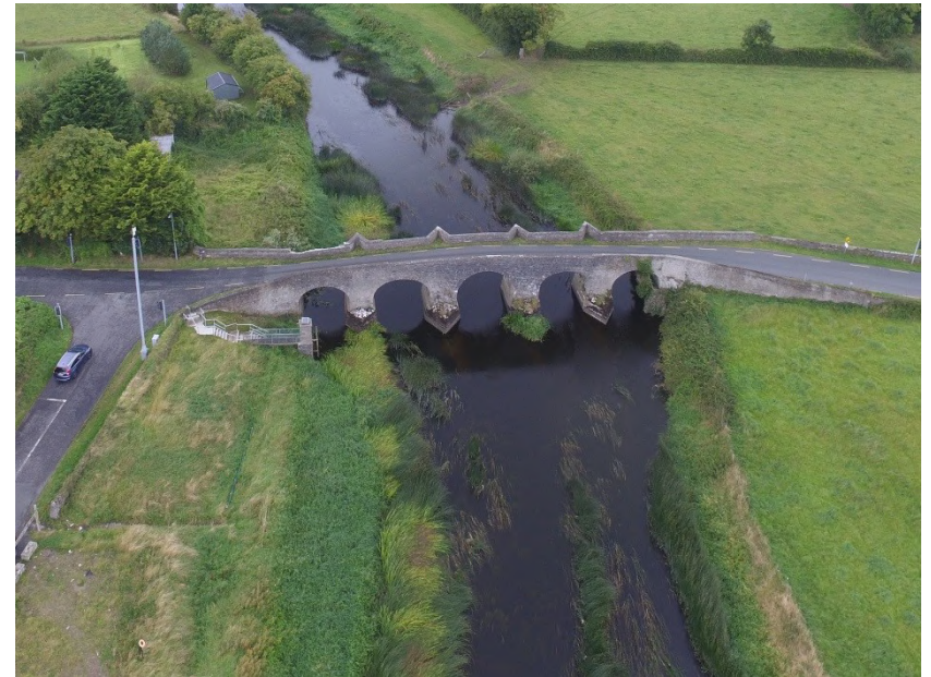
Plate 2: General view of Pass Bridge, looking north
