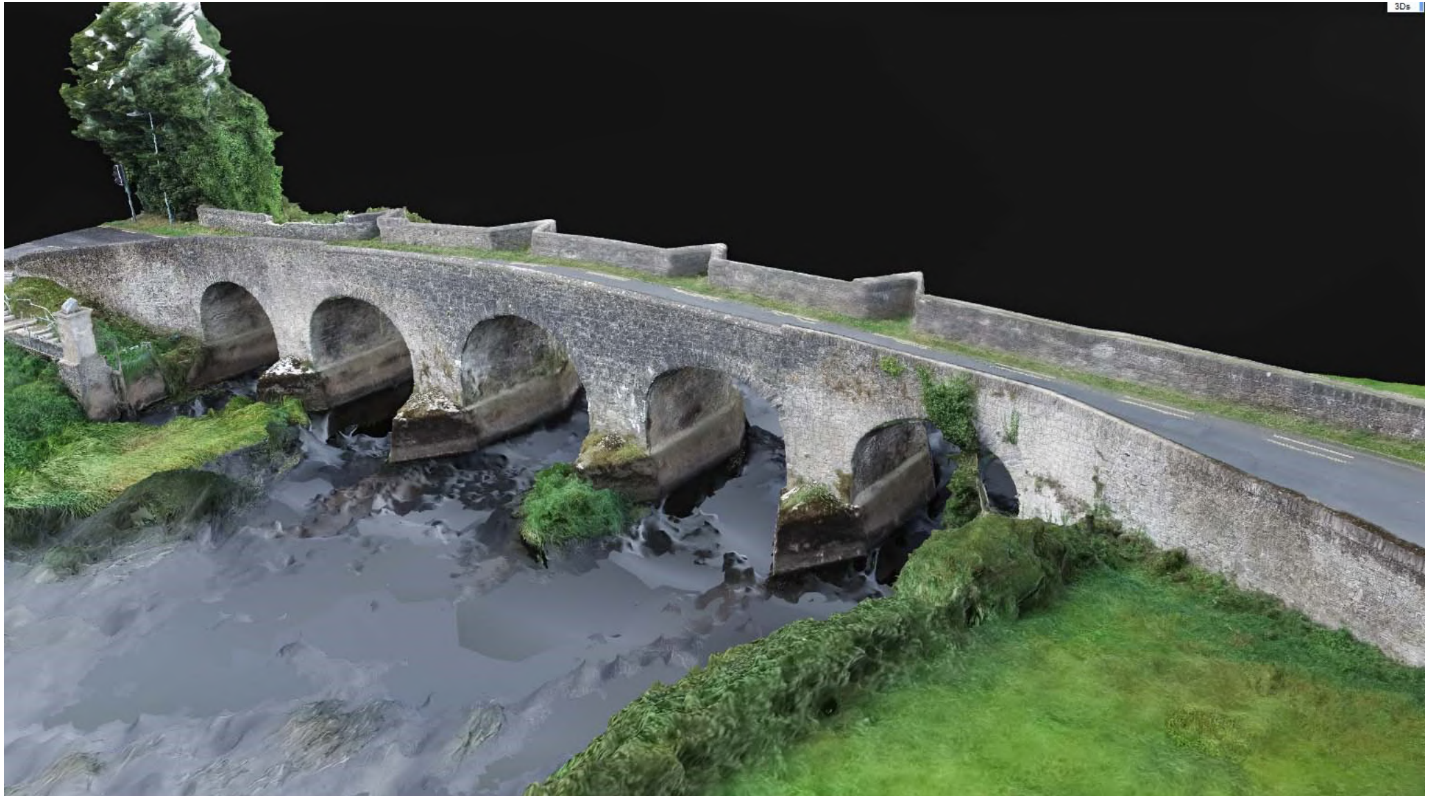
Plate 13: South-facing elevation, oblique view looking northwest
