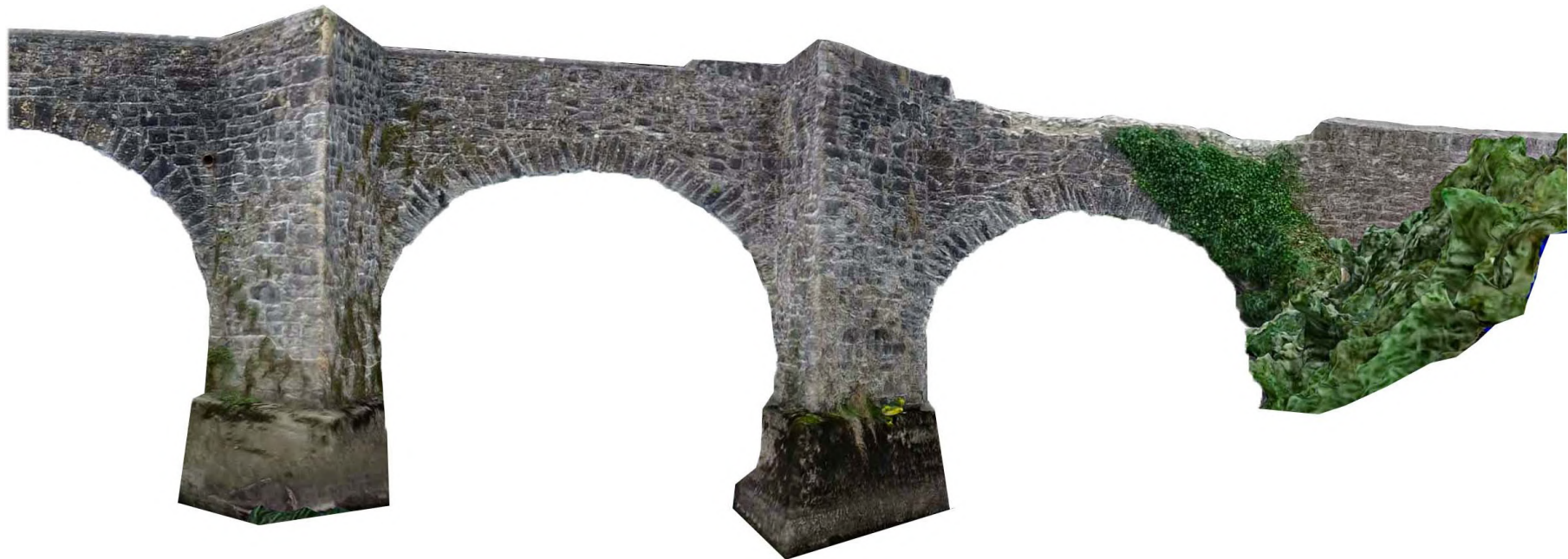
Plate 7: Detail of north-facing elevation, west side
