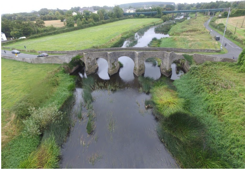
Plate 1: General view of Pass Bridge, looking south, with Barrow Bridge visible in background
