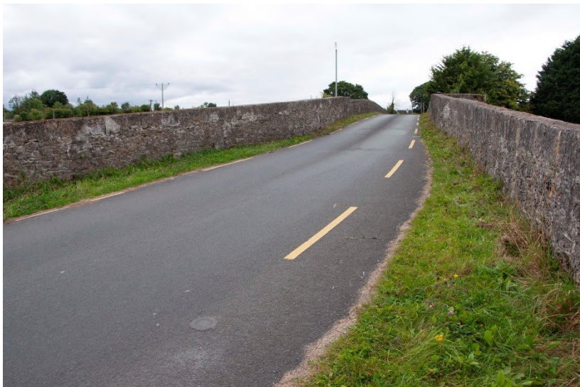
Plate 28: Approach walls on east side of bridge, looking southwest
