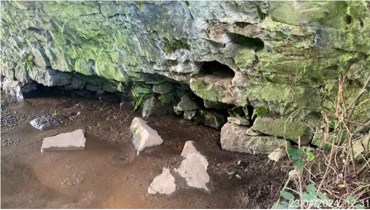
PHOTO 04 RELIEF ARCH UNDERMINING / COLLAPSED ABUTMENT
