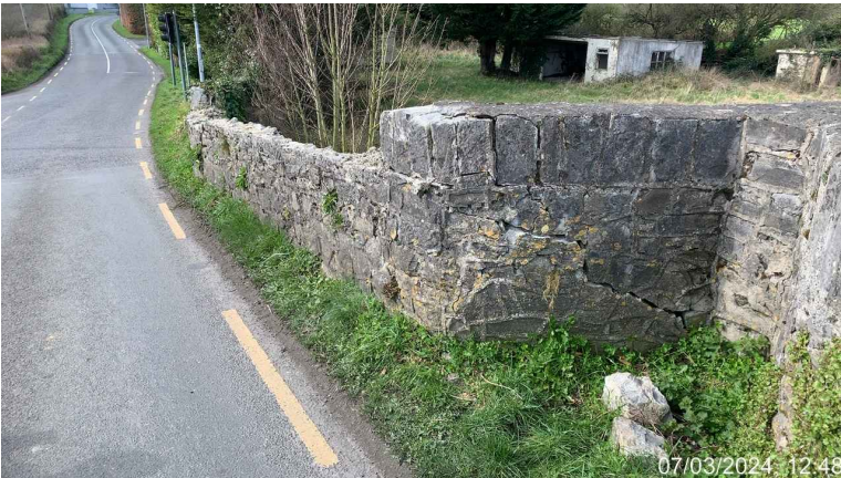
PHOTO 02 UPSTREAM SPAN 1 DAMAGED PARAPET
