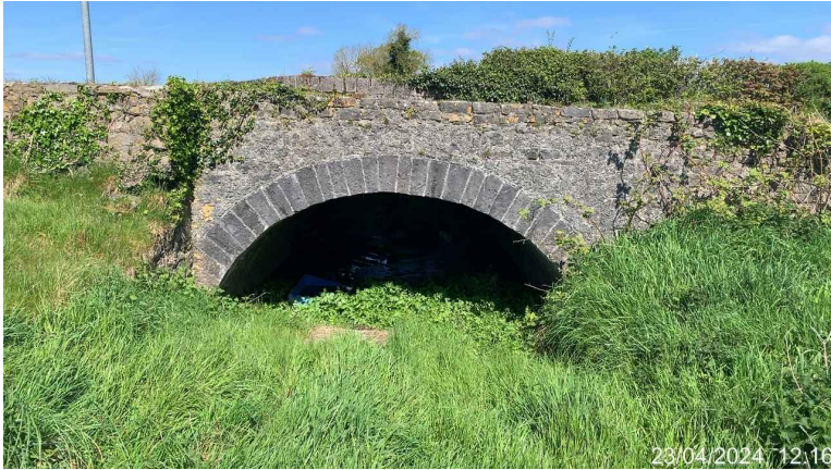
PHOTO 09 RELIEF ARCH DOWNSTREAM
