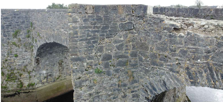
PHOTO 03 UPSTREAM SPAN 1 DAMAGED CUTWATER/CRACKING
