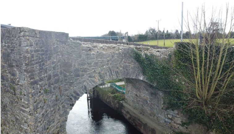
PHOTO 01 UPSTREAM SPAN 1 MISSING COPING
