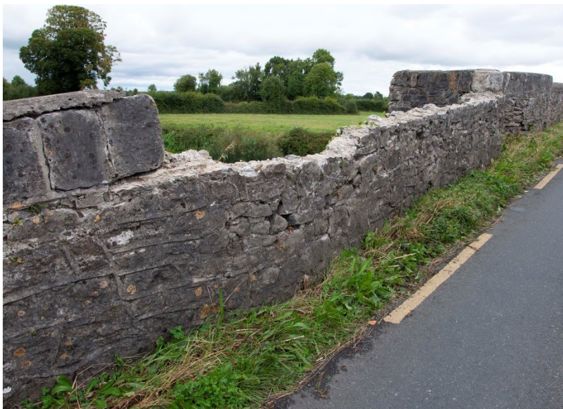
Plate 26: Detail of recent damage to north approach wall on west side of bridge
