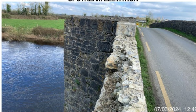
PHOTO 2 (MISSING PARAPET COPING AND CUTWATER CRACKING)
