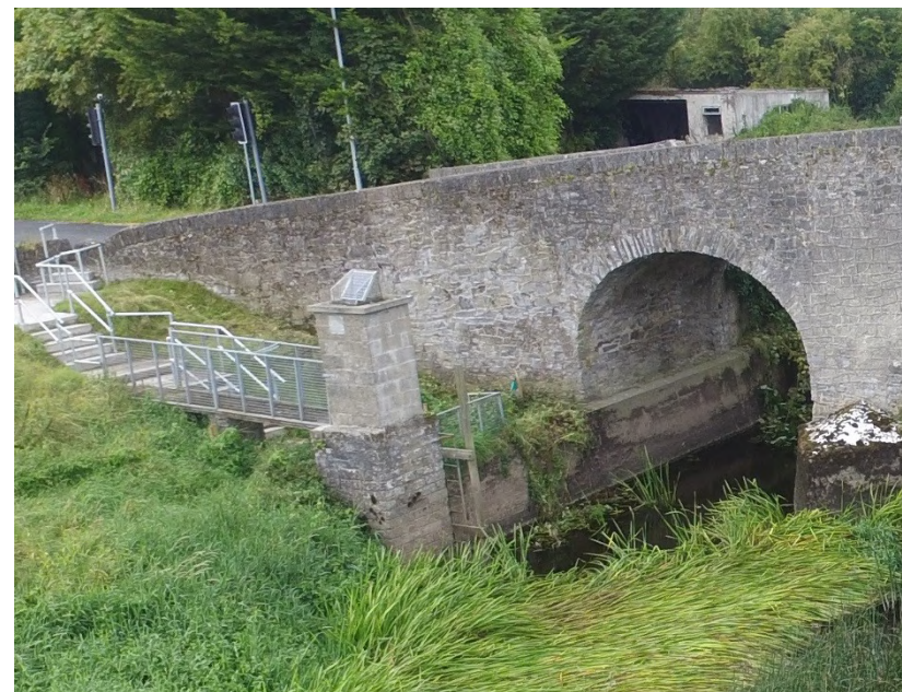
Plate 21: Detail of abutment and side wall on west side of south-facing elevation
