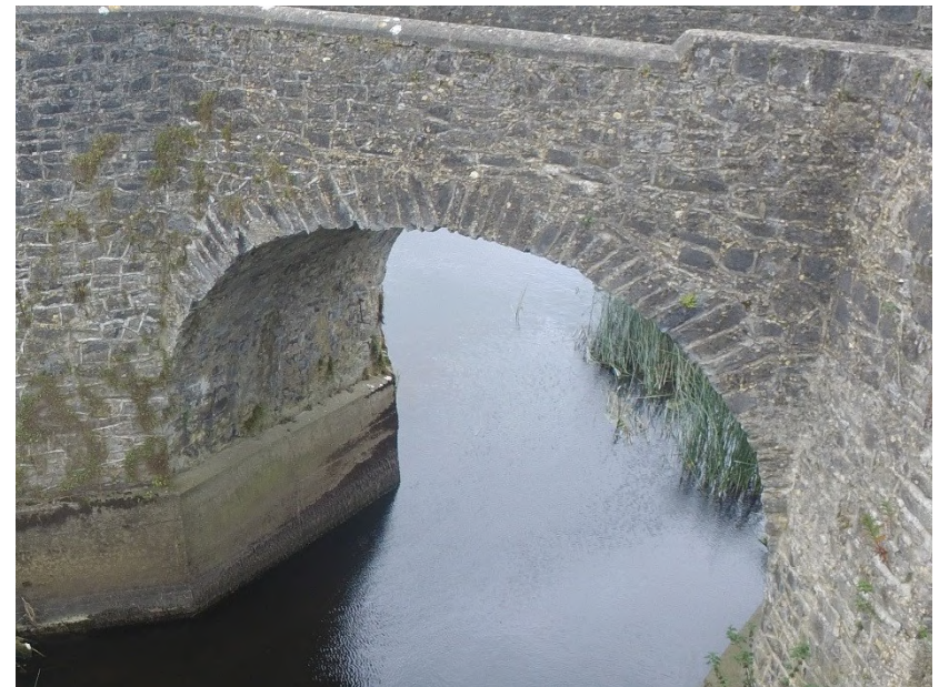
Plate 17: Detail of voussoirs on north-facing elevation
