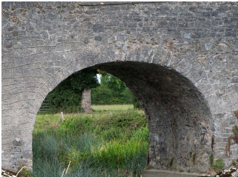
Plate 18: Detail of voussoirs on south-facing elevation, with rendered soffit visible
