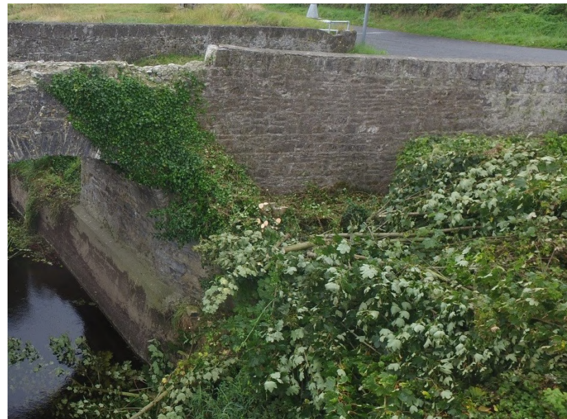
Plate 19: Detail of abutment and side wall on west side of north-facing elevation
