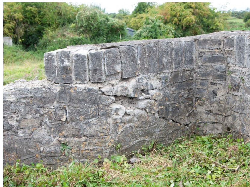
Plate 27: Cracking visible in triangular cut-water in north wall on west side of bridge
