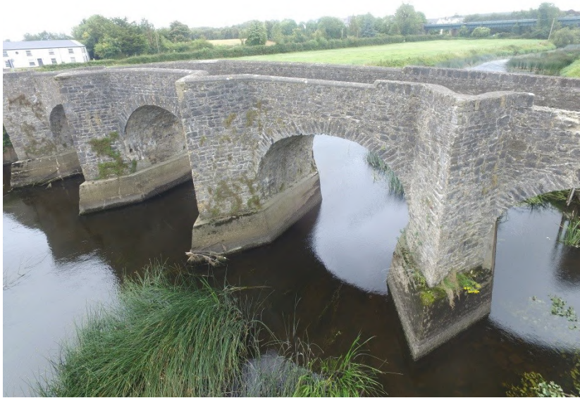
Plate 14: View of triangular cut-waters on north-facing elevation
