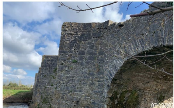
PHOTO 3 (CUTWATER CRACKING)
