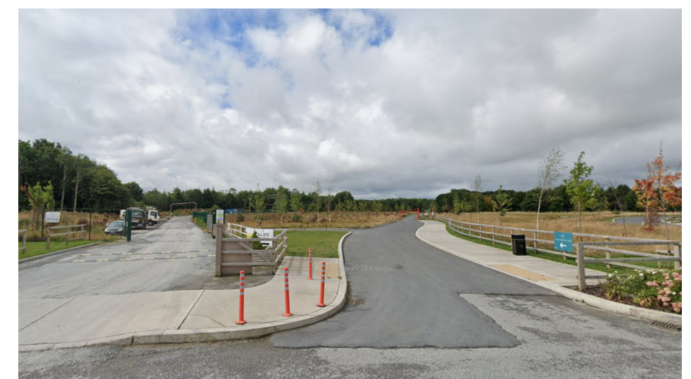
Figure 20: Main entrance into the site.
