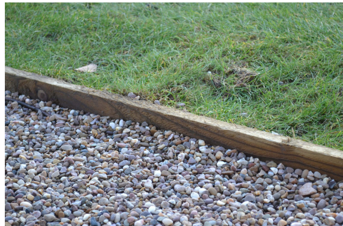
Loose gravel & timber edge - Allotments
