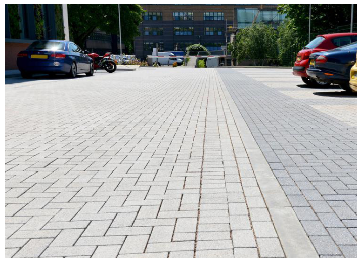
Hydropave to parking bays
