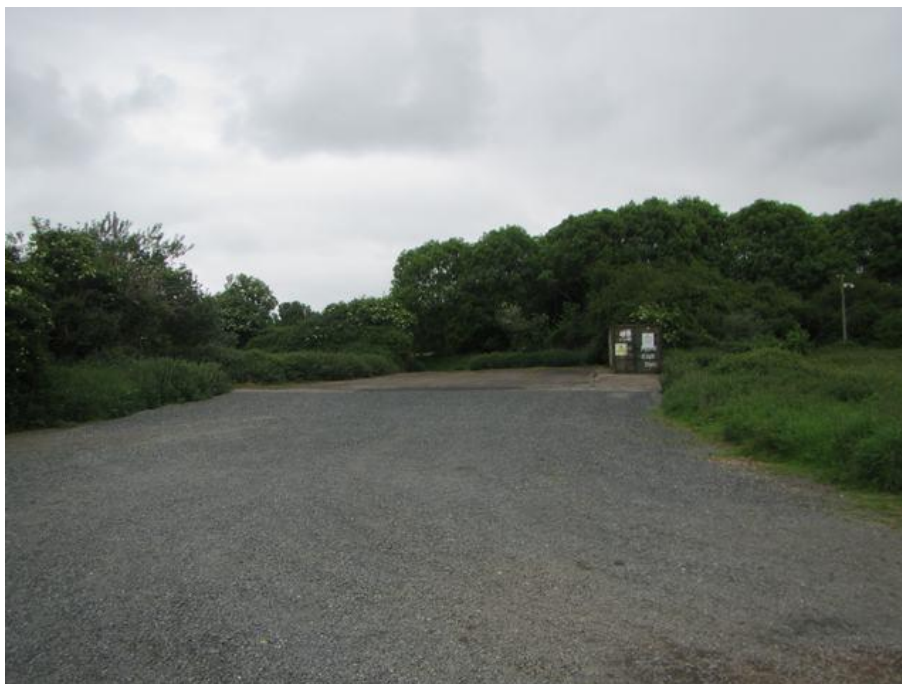
Plate 13 Concreted area to the north of the access road where the new 174sqm building will be located.
