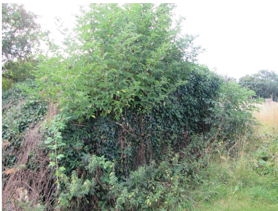
Plate 16 Overgrown wall at the southeast of the laneway.
