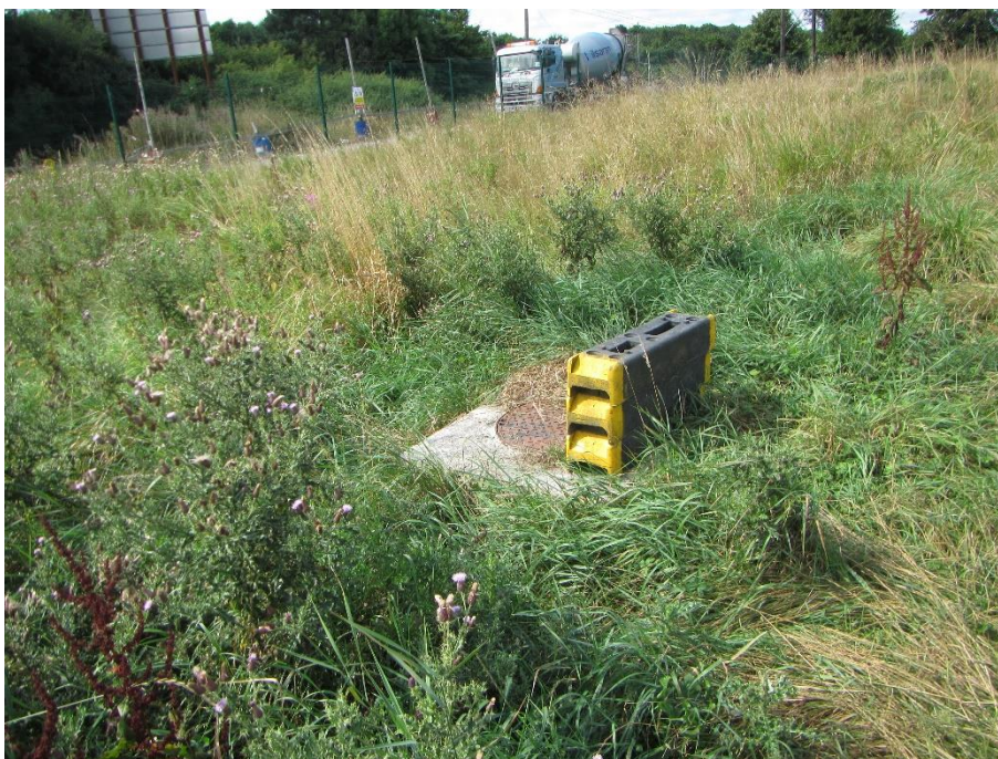
Plate 19 Manhole within the triangular field.
