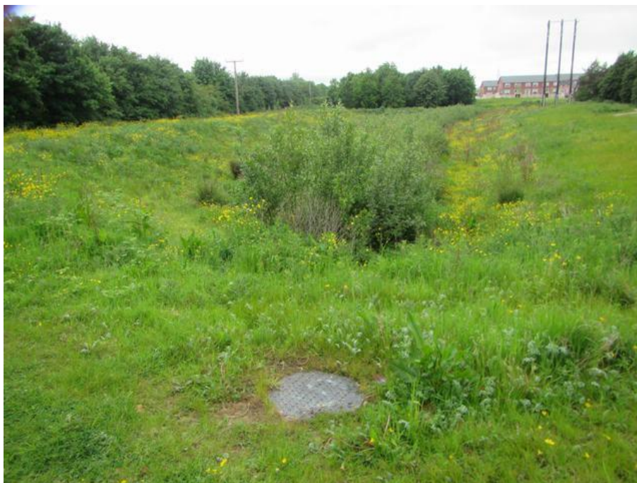
Plate 20 Modern attenuation area and drainage installed during the last two years.
