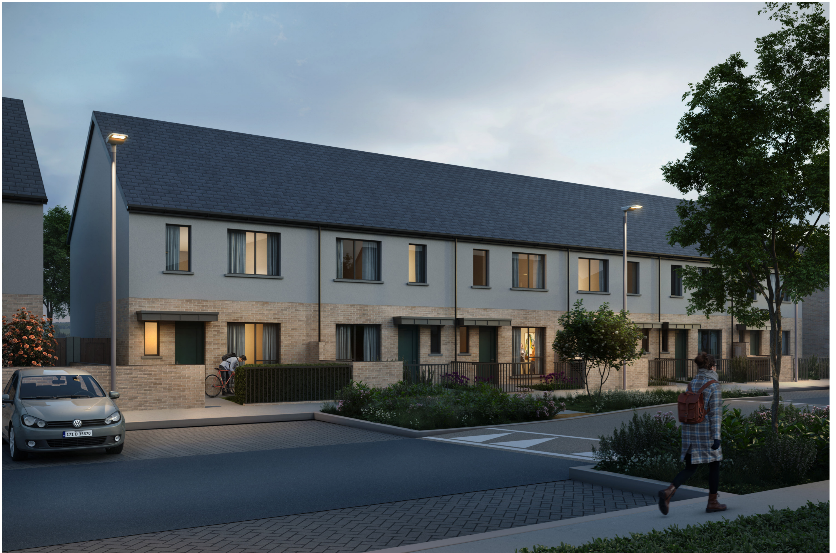
Image 27: View along central street of two-bed terrace
