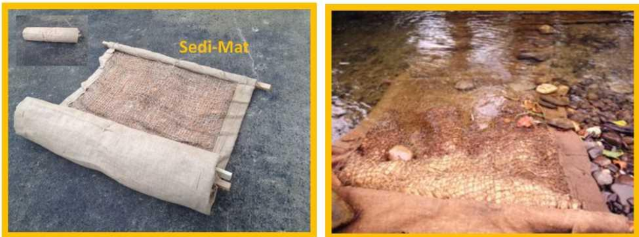
Fig 2.2. An example of the sedimat to be placed in near waterways before the commencement of works on site.
