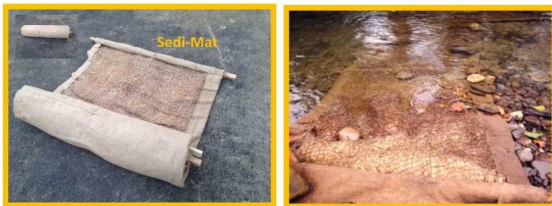
Fig 2.3. An example of the sedimat to be placed near waterways before the commencement of works on site.
