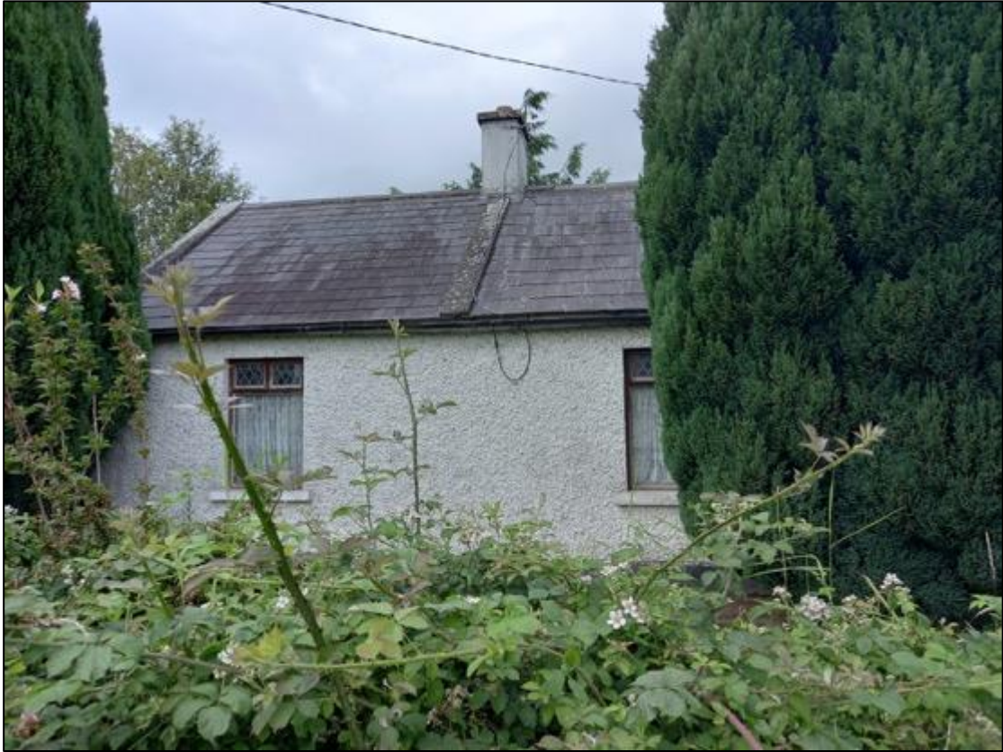
Plate 2.1 – Dwelling house and hedgerow habitats present in application site .
