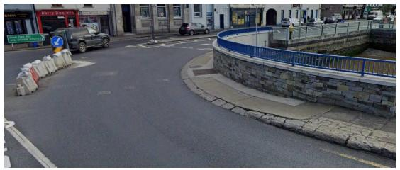
Plate 6-3 Broken Kerbs and Footway are Evidence of Commercial Vehicle Overrun
