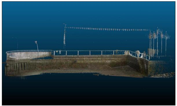
Plate 14.13 LiDAR scan elevation of masonry quay wall, flood relief wall and steps, facing east
