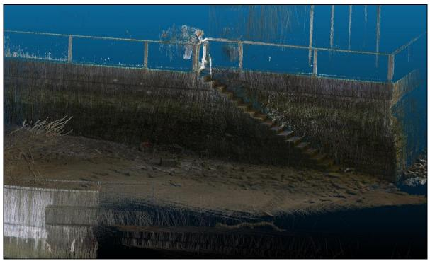
Plate 14.14 LiDAR scan elevation of masonry quay wall and steps, facing southeast
