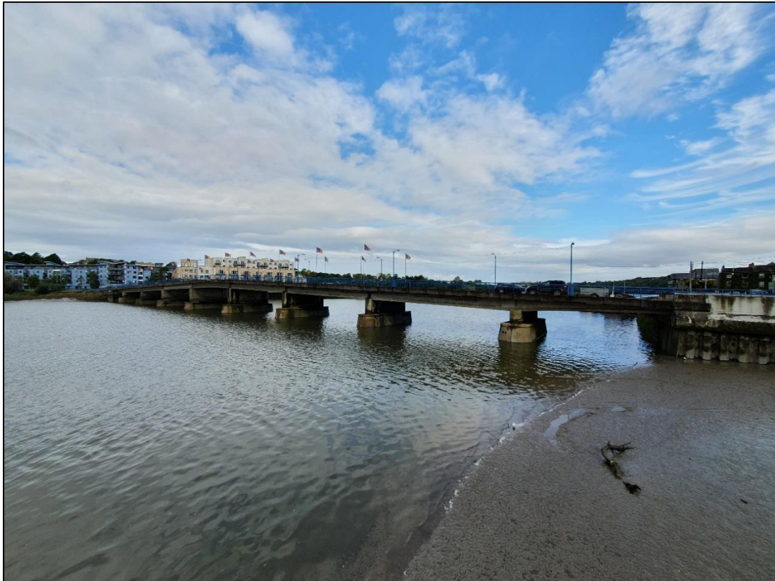
Plate 2-7 Estuary / Tidal River flowing under O'Hanrahan Bridge.
