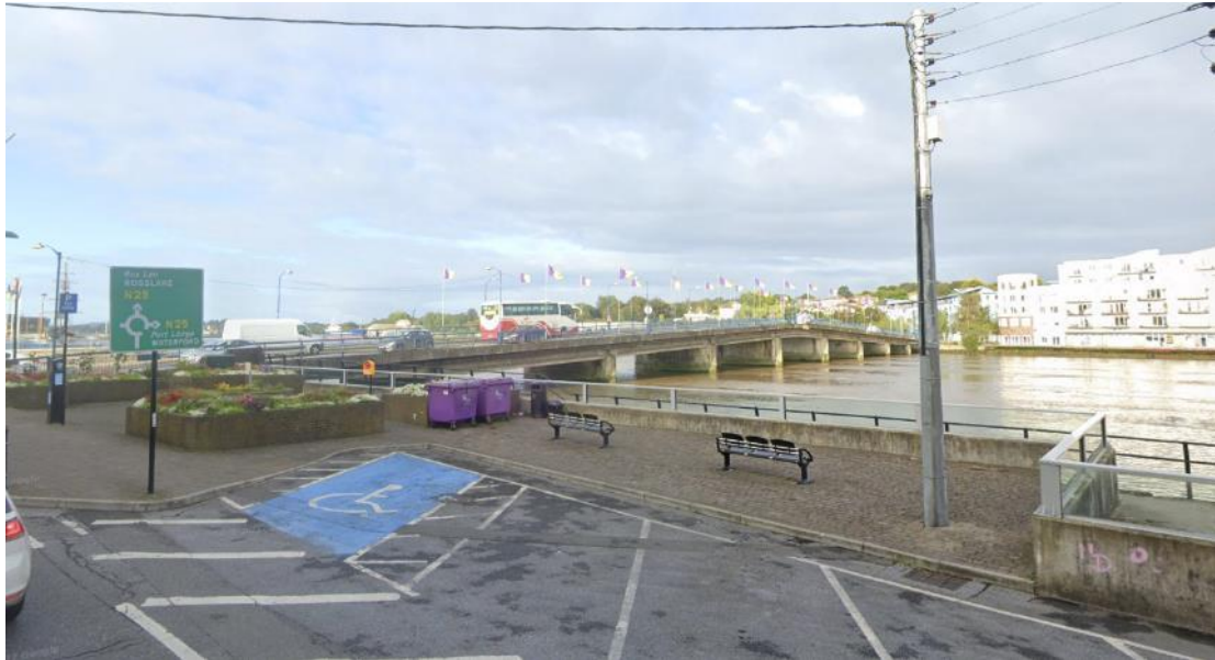
Plate 2.4 New Ross Quay with views to the south. In the foreground are the existing road, parking spaces, existing flood defence wall and a public realm consisting of a small square with benches and flower beds. In the background is the O'Hanrahan Bridge and the Rosbercon Quay. © Google Street View
