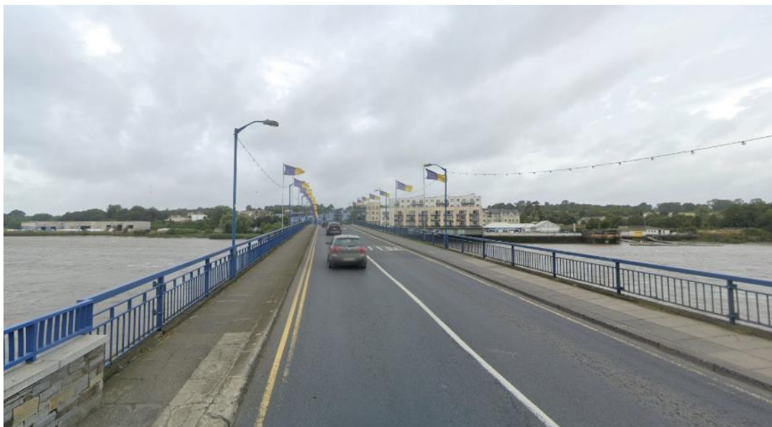
Plate 2.3 O'Hanrahan Bridge with view to the north-west. In the foreground are the existing road of the bridge and the narrow footpaths along the sides that are proposed to be widened as part of the development. The existing parapets are proposed to be replaced. © Google Street View
