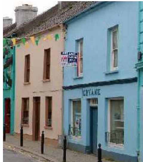
Fig. 86 - Examples of Modest shop front approach in Dingle Co. Kerry, utilising window and door openings positioned with consideration to the existing first floor windows, and their proportions, with simple signage demarcating the commercial activity. This example is an appropriate approach for commercial uses on the northern side, and at the western end of Claregate Street.
