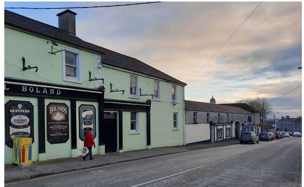
Fig. 59 - View From Bride Street Towards Market Square
