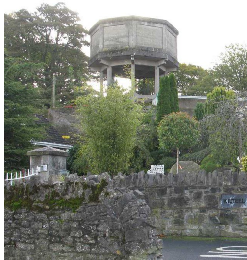
Fig. 51 - View Of Water Tower From Nugent Street
