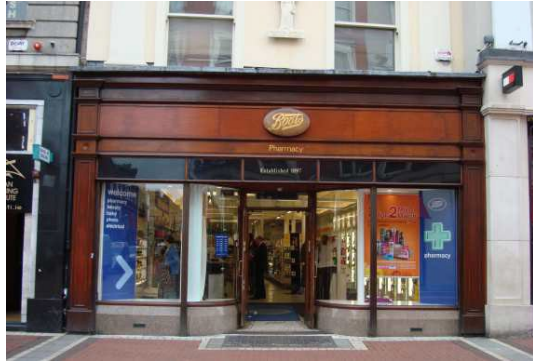
Fig. 83 - Boots Grafton Street, Dublin Example of Corporate Shopfront with discreet signage.
