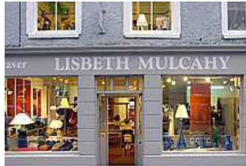
Fig. 85 - Examples of contemporary shop front, well proportioned windows, and the simple use of render as the shop front, render fascia and signage over, and use of subtle colour palette. This example is an appropriate approach for commercial uses on Bride Street and Claregate Street, between the Market Square and Bang Up Lane. This approach is also suitable for a number of properties on Market Square.
