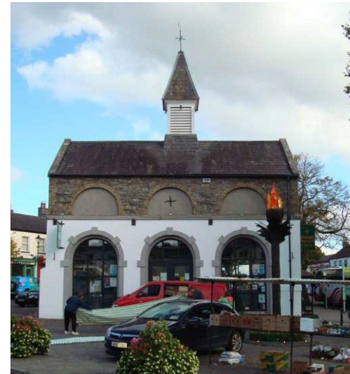
Fig. 25 - Market Building Kildare Town
