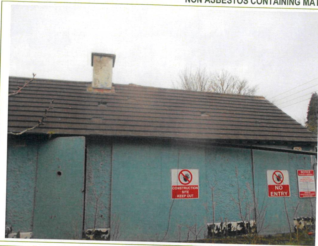
Concrete roof tiles
