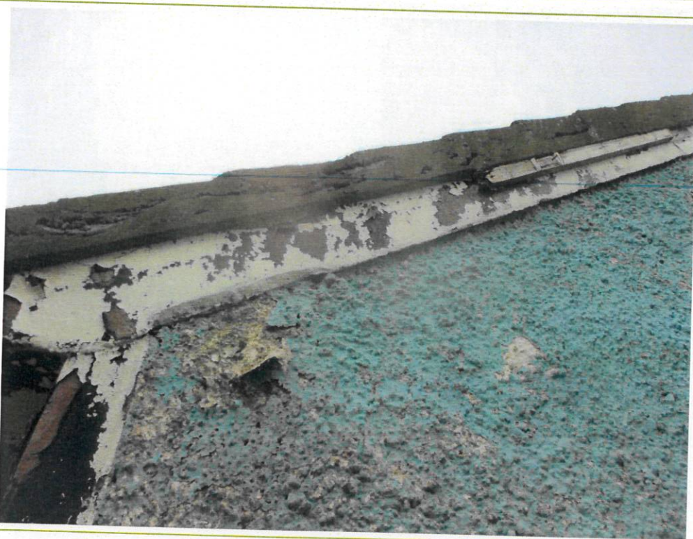
roof barge to front of property
