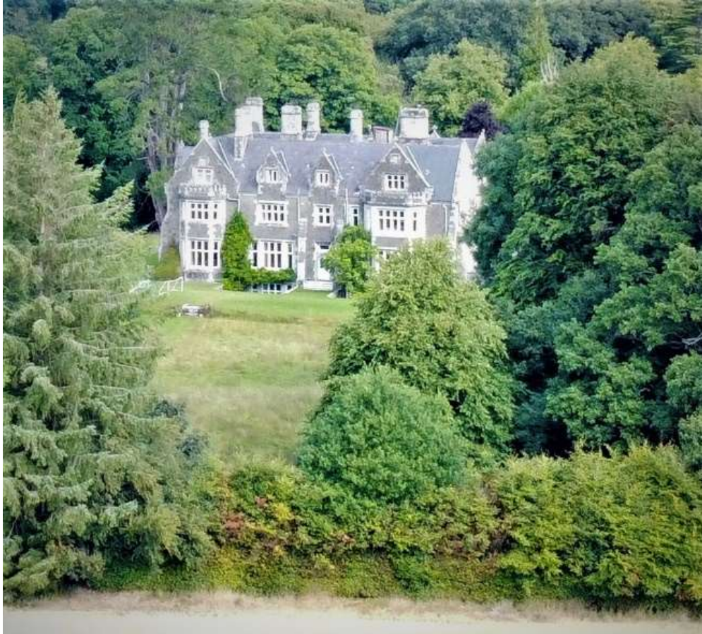
Fig. 6 – Image of the south facing façade (taken 2022)
