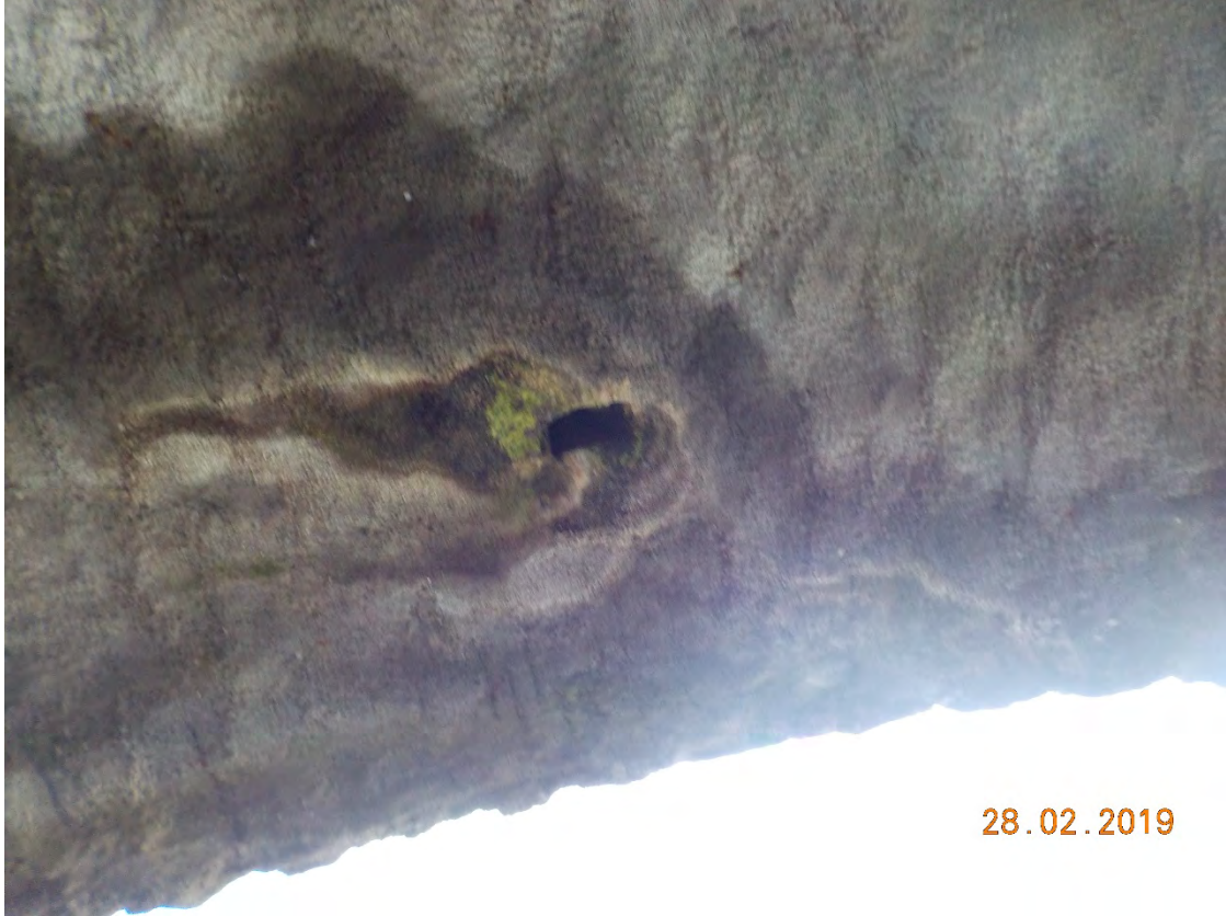
Photograph 3-65: Arch 4 – Bridge Deck
