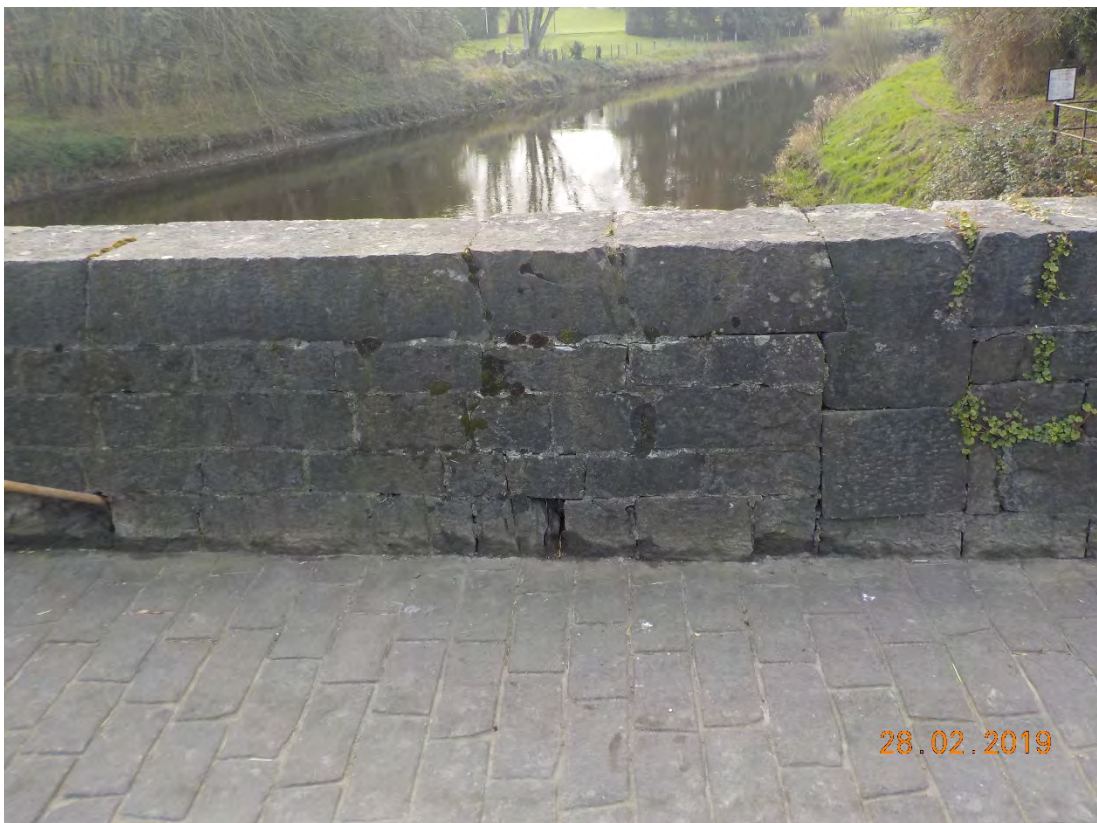
Photograph 3-20: Section of Wall to be reconstructed on the Downstream Side
