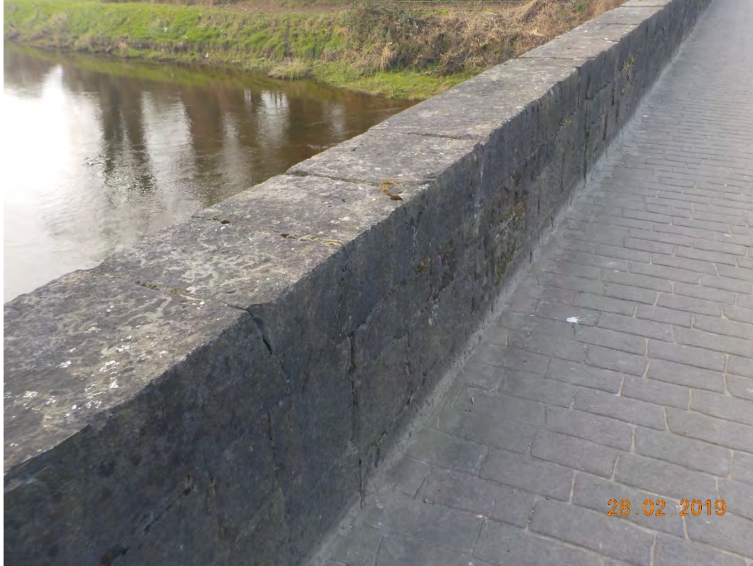
Photograph 3-17: Rake and Repoint joints in Downstream Road side Parapet
