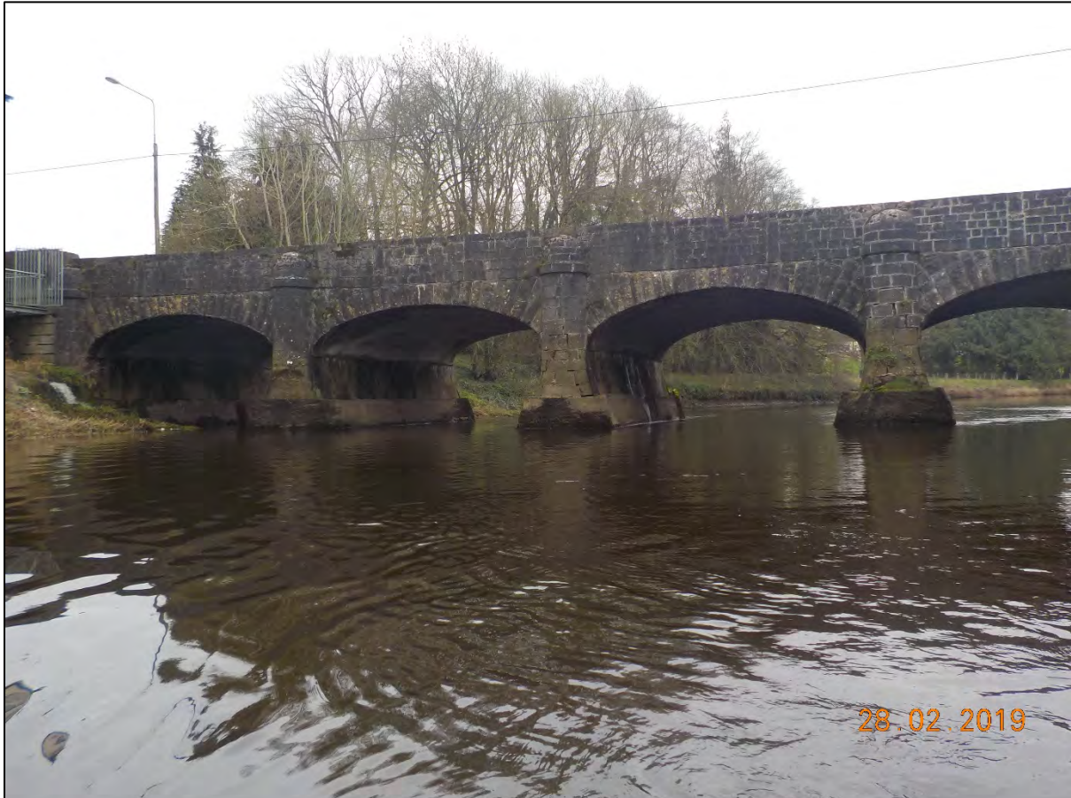
MONASTEREVIN BRIDGE UPSTREAM FACE
