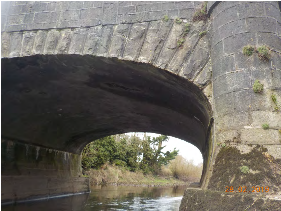
Photograph 3-59: Pier 2 – Spandrel Walls
