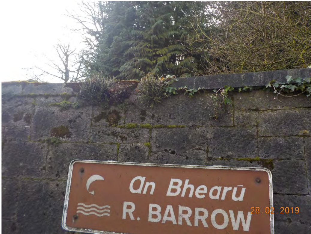
Photograph 3-5: Downstream Capping on Road Side Parapet
