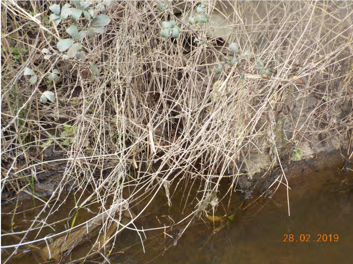
Photograph 3-38: Downstream Left Embankment Retaining Wall
