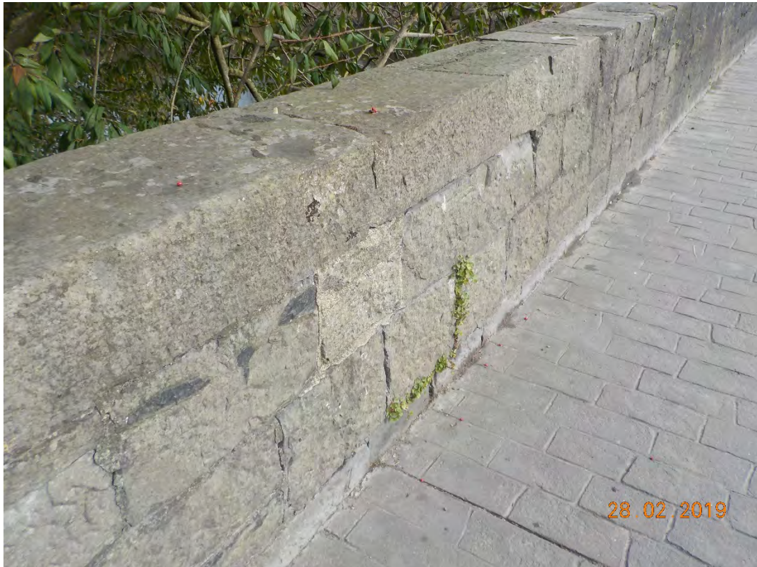
Photograph 3-29: Upstream Roadside Parapet Wall
