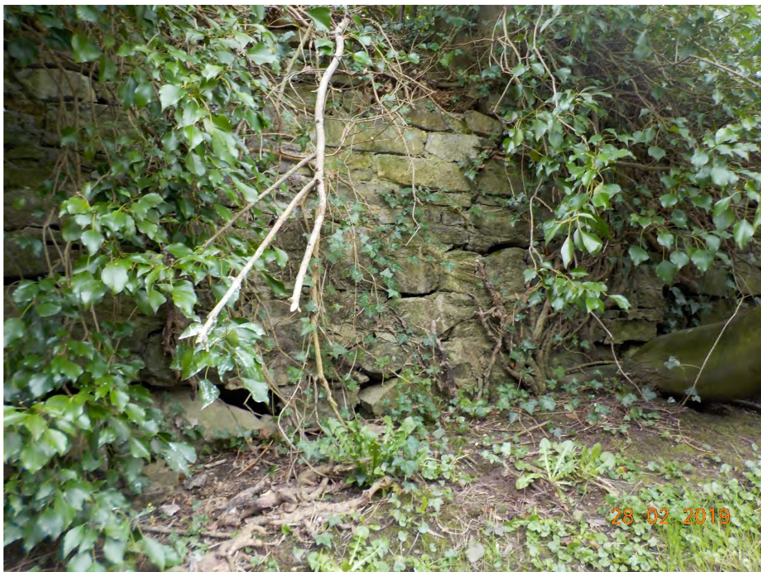
Photograph 3-77: Retaining Wall to be reconstructed
