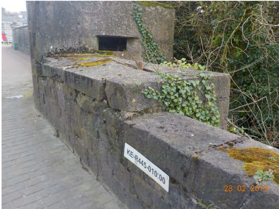
Photograph 3-9: Downstream roadside West Parapet
