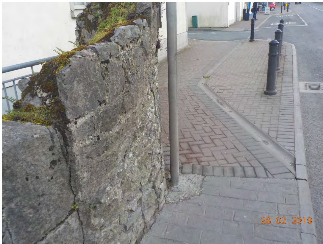
Photograph 3-34: Upstream Roadside Parapet Wall
