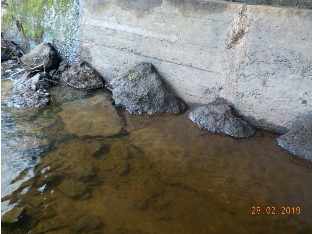
Photograph 3-76: River Bed under Arch 5
