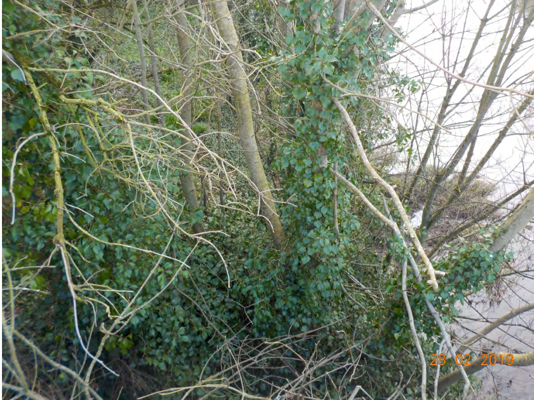
Photograph 3-37: Remove Tree's on Downstream Left Embankment
