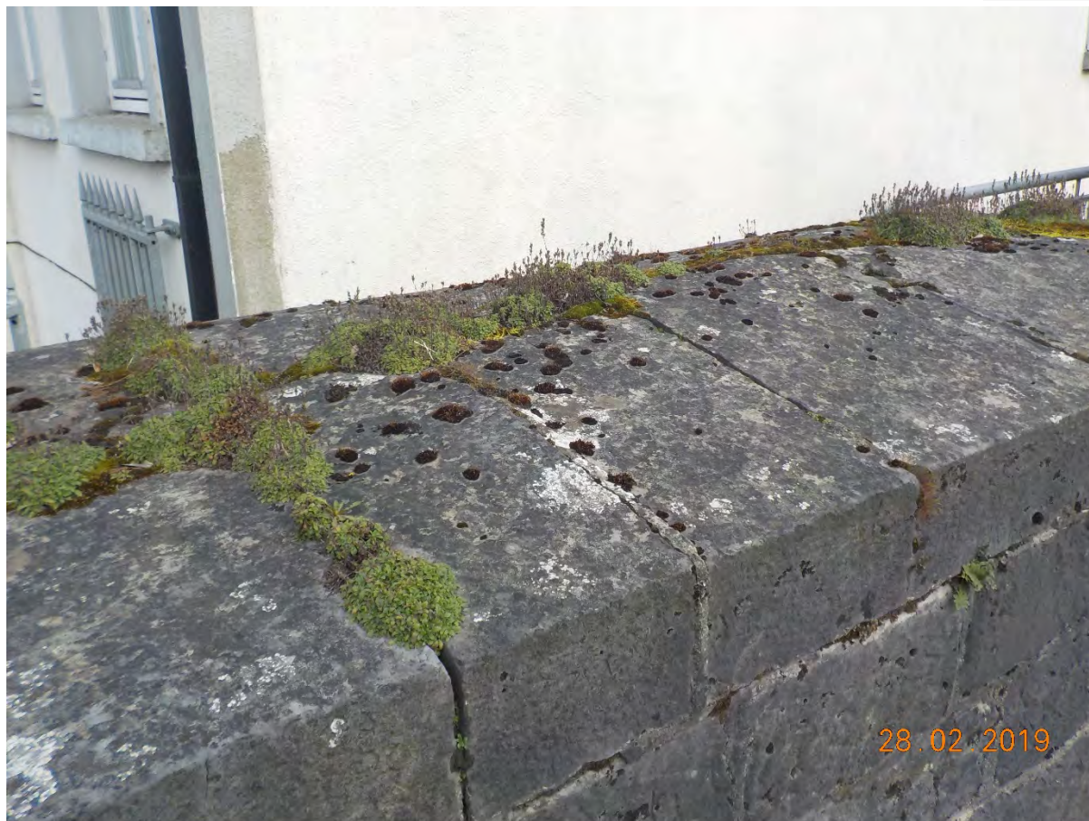
Photograph 3-31: Capping on Upstream Roadside Parapet
