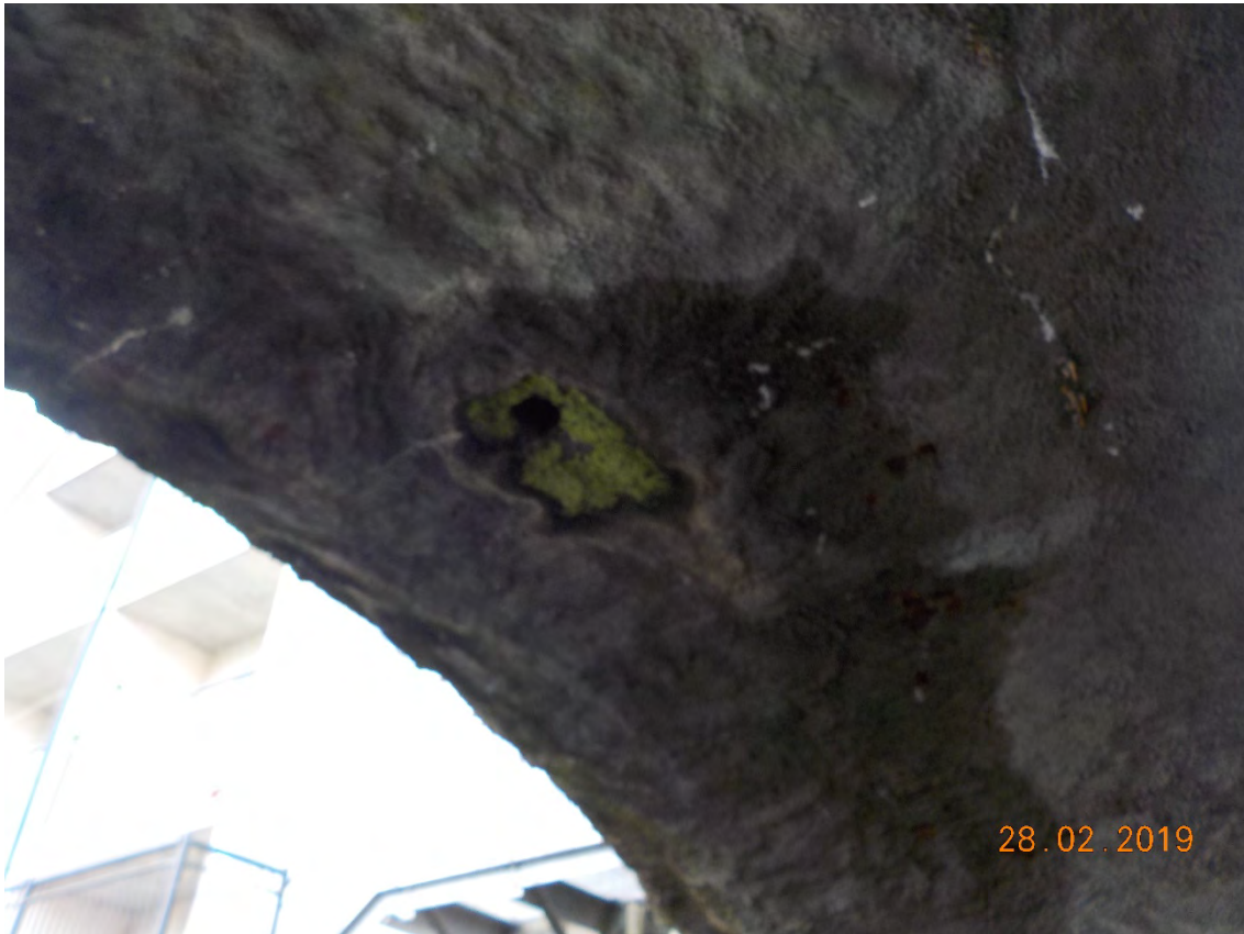
Photograph 3-72: Arch 5 Decking Upstream
