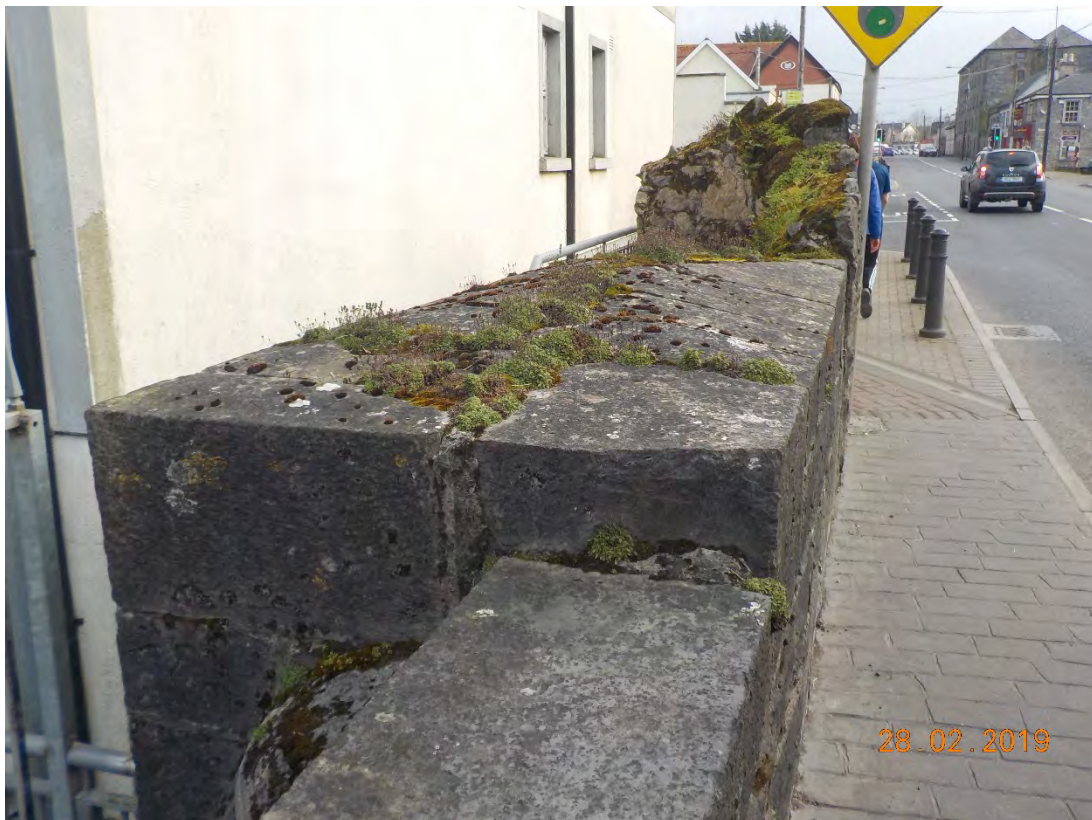
Photograph 3-30: Capping on Upstream Roadside Parapet
