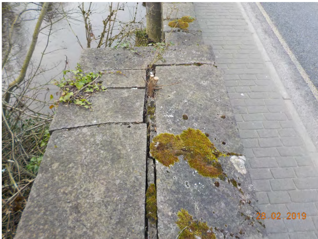
Photograph 3-10: Downstream Parapet Roadside Approach
