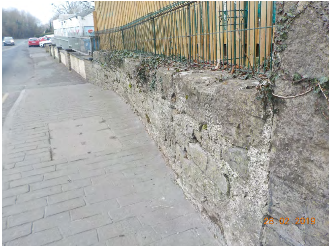
Photograph 3-27: Vegetation on Upstream side Parapet Capping.
