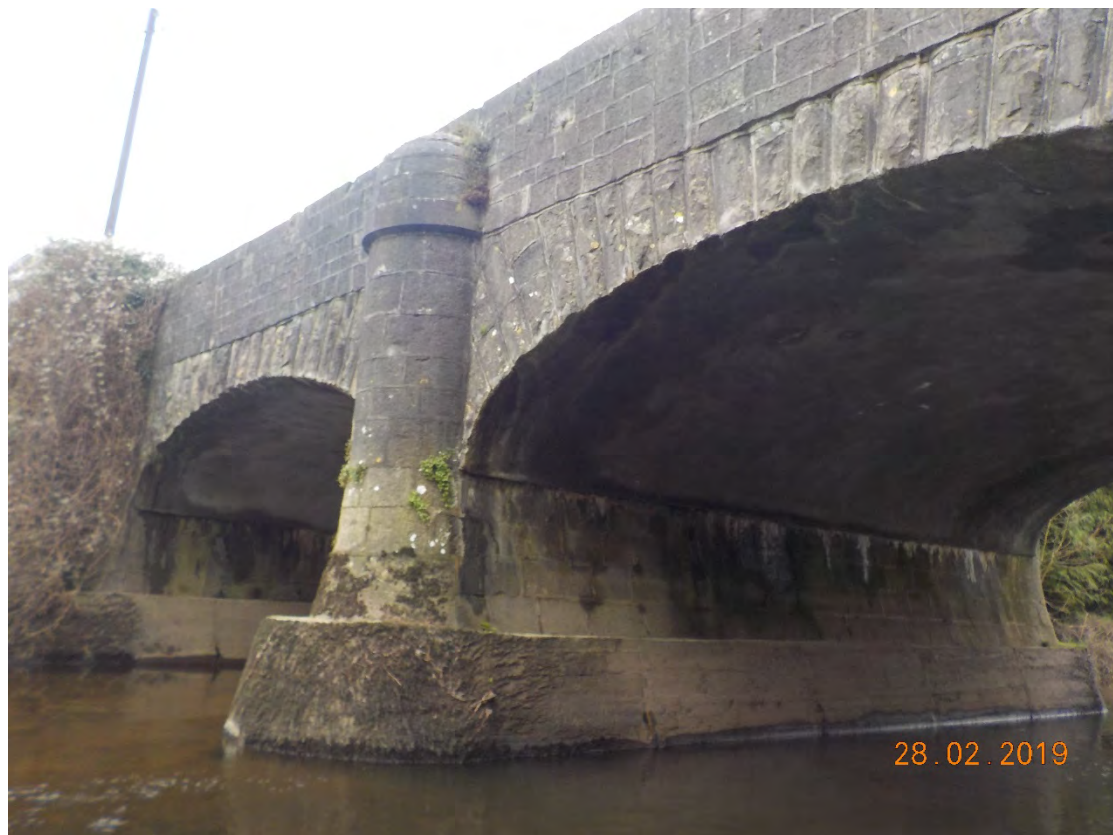
Photograph 3-60: Pier 2 – Spandrel Walls
