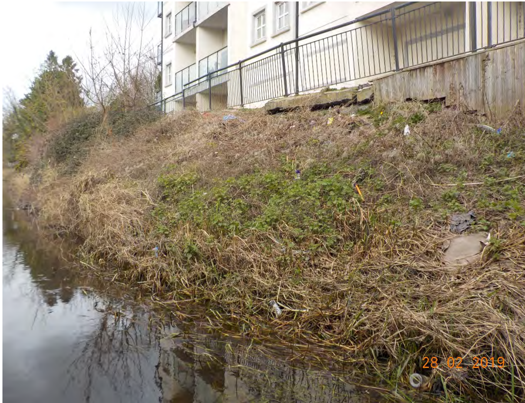
Photograph 3-47: Upstream East Embankment
