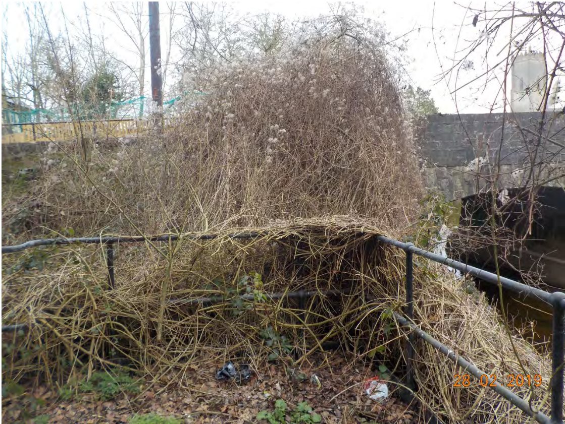
Photograph 3-43: Tree's to be removed on Downstream Left Embankment
