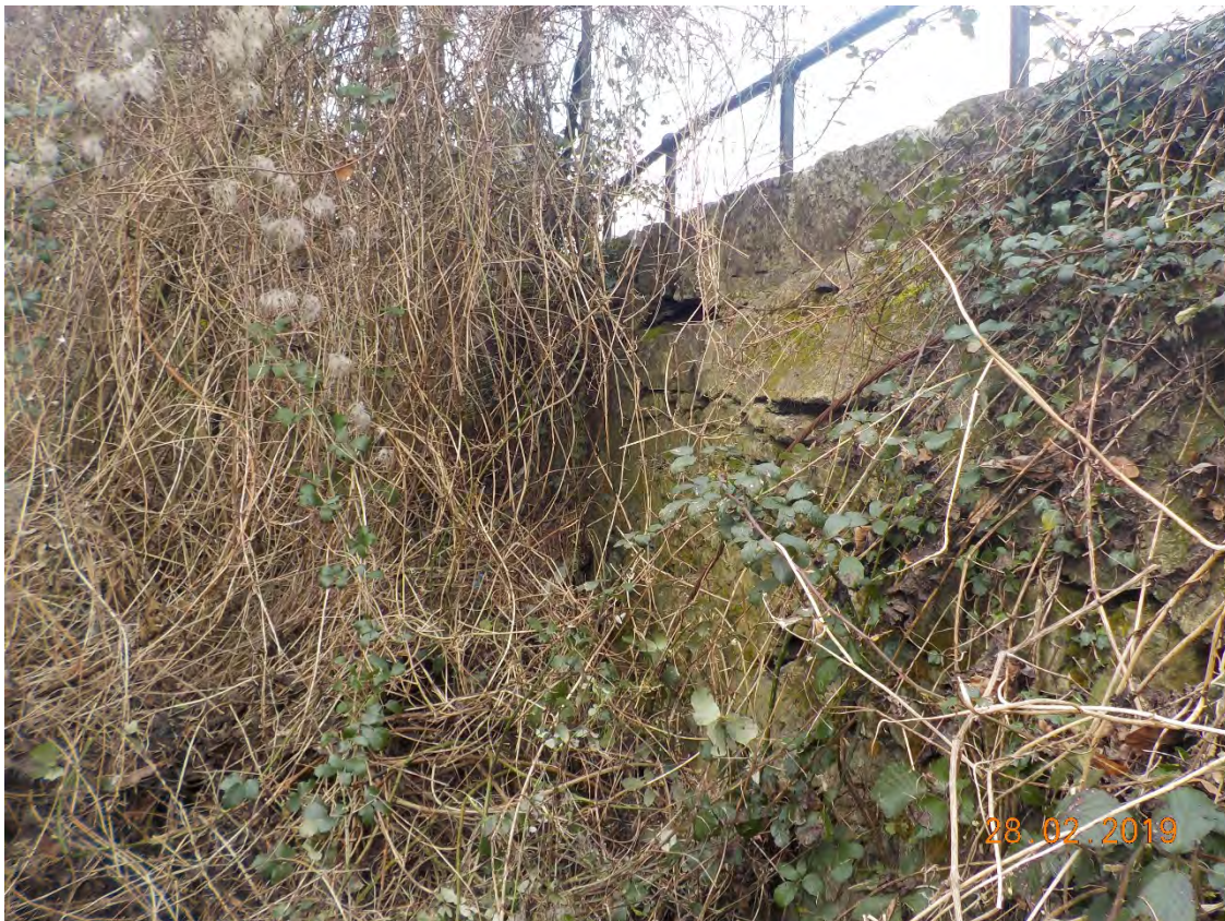
Photograph 3-44: Downstream Riverside Parapet
