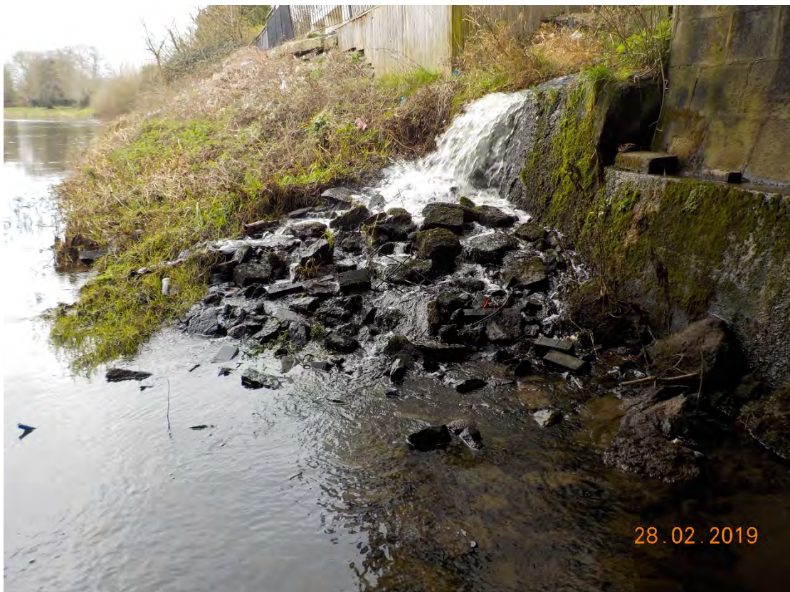
Photograph 3-75: River bed under Arch 5
