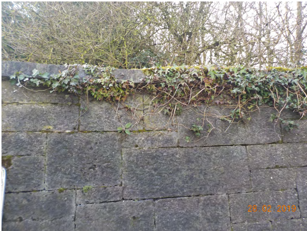
Photograph 3-6: Downstream Capping on Road Side Parapet
