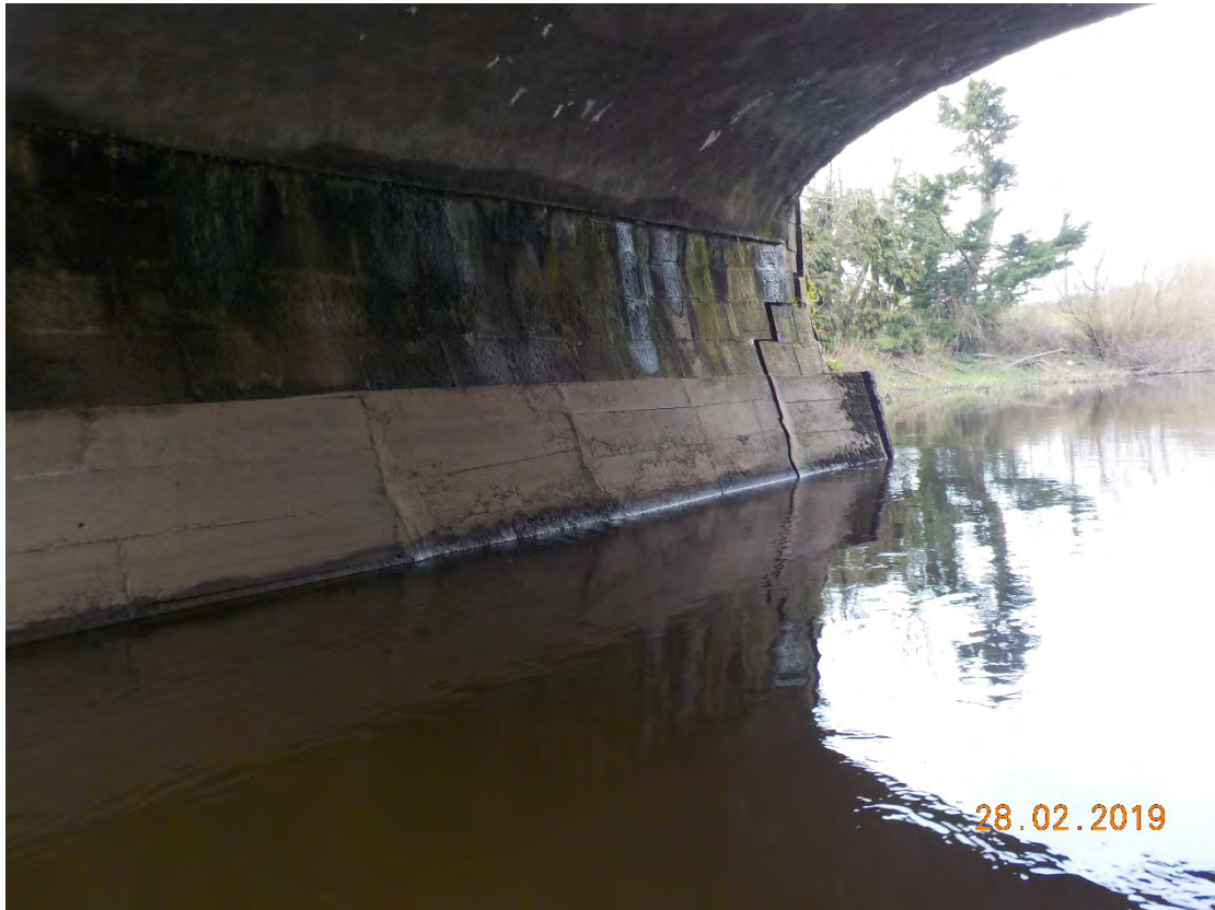
Photograph 3-61: Arch 3 – West Abutment
