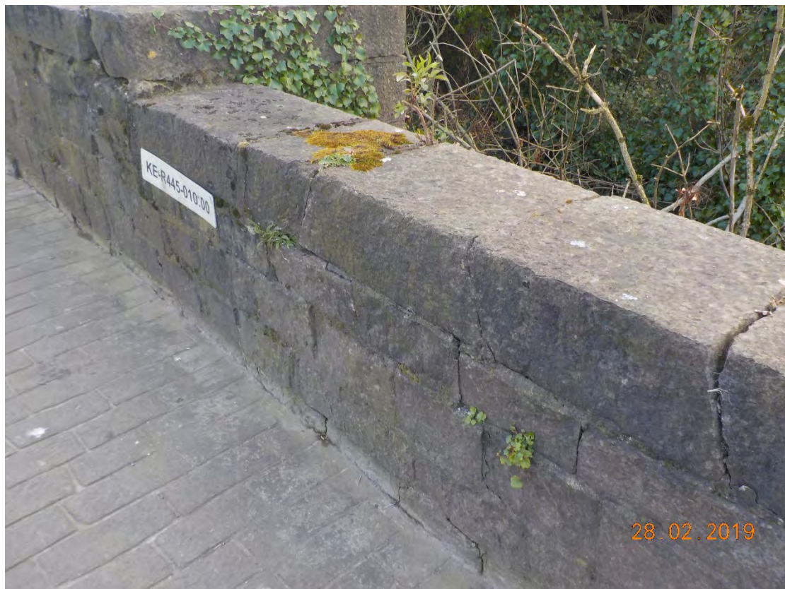
Photograph 3-16: Rake and Repoint joints in Downstream Road side Parapet
