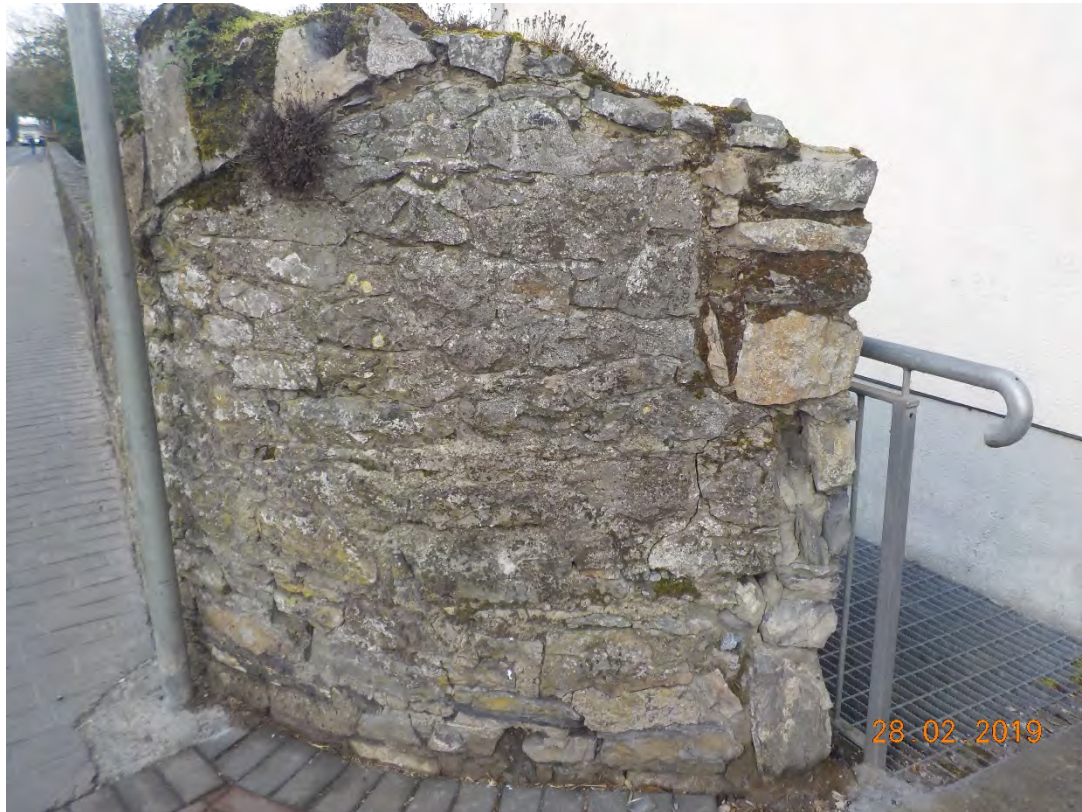
Photograph 3-33: Upstream Roadside Parapet Wall
