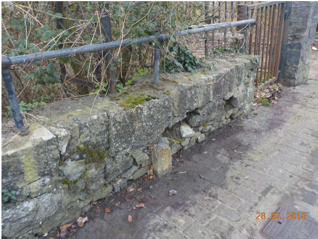
Photograph 3-26: Wall to be reconstructed on downstream side
