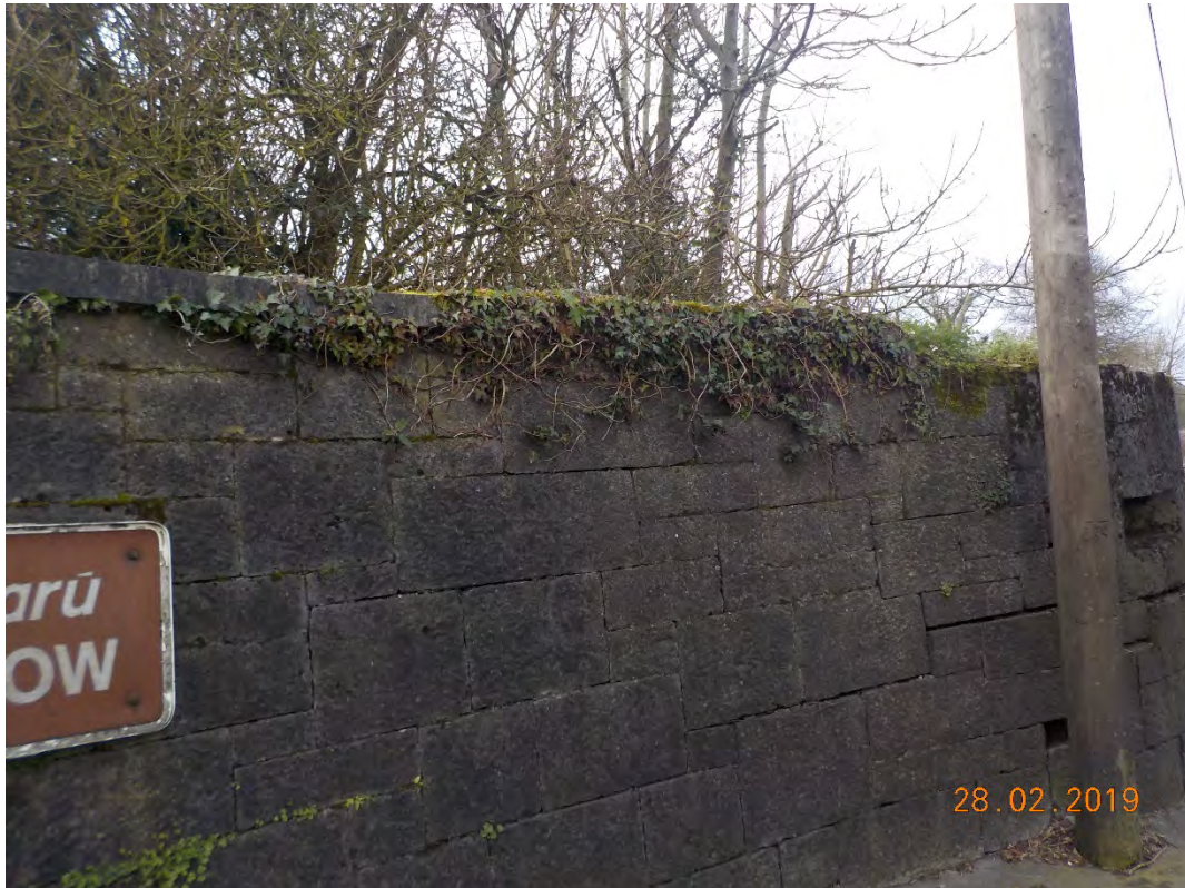
Photograph 3-7: Downstream Capping on Road Side Parapet
