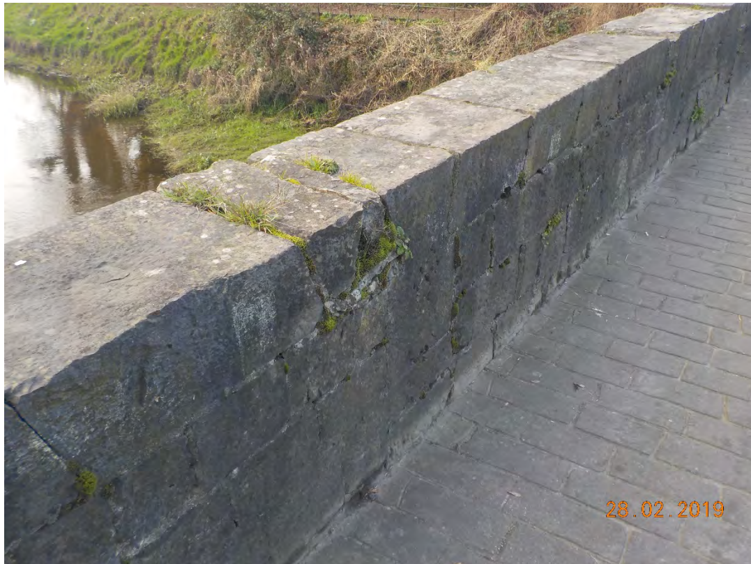
Photograph 3-18: Rake and Repoint Joints in Downstream Road Side Parapet
