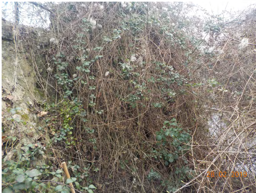
Photograph 3-45: Downstream Riverside Parapet
