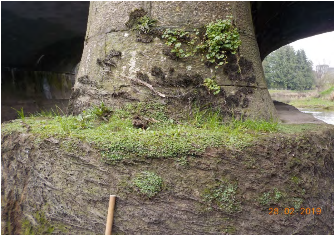
Photograph 3-53: Pier 1 – Rake and Repoint
