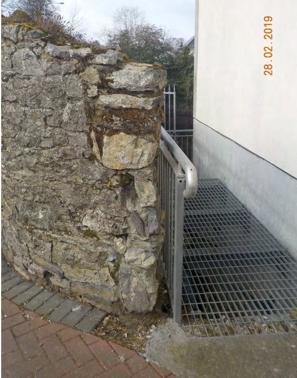
Photograph 3-32: Upstream Roadside Parapet Wall
