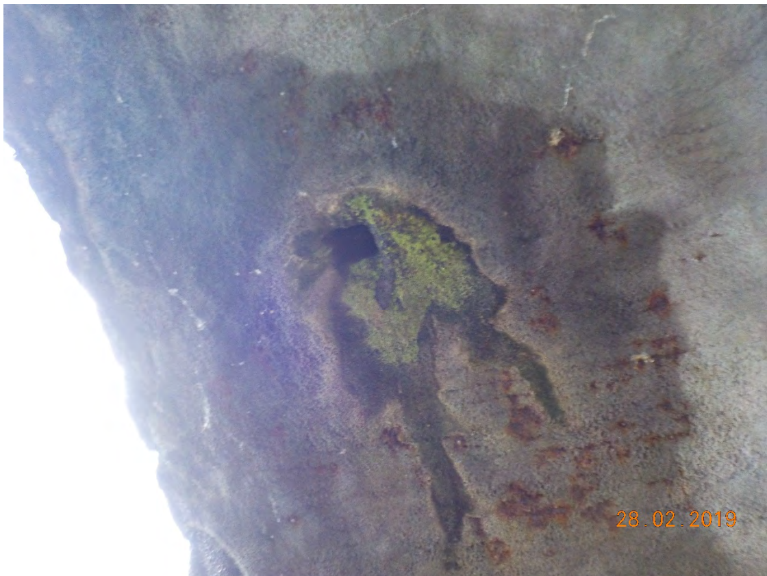
Photograph 3-64: Arch 4 - Bridge Deck
