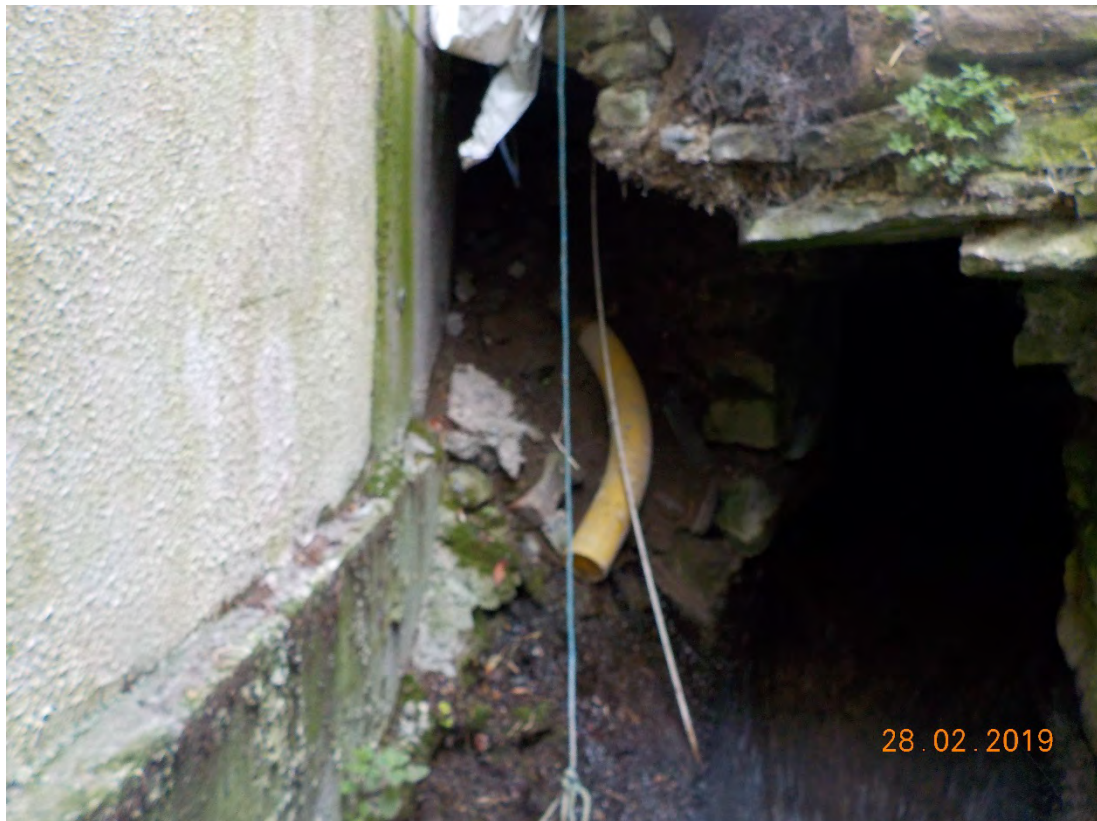
Photograph 3-50: Wall to be reconstructed
