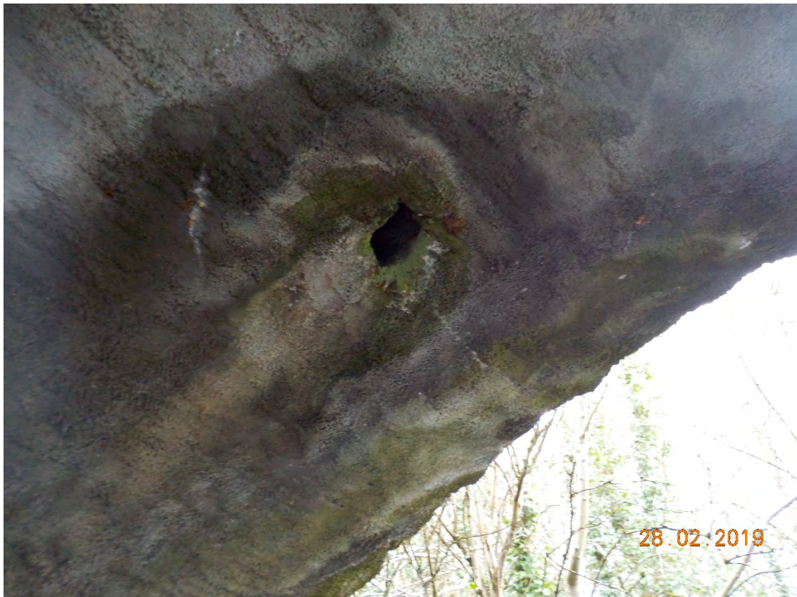
Photograph 3-73: Arch 5 Decking Downstream
