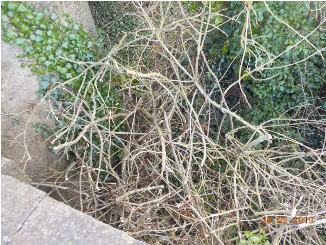
Photograph 3-35: Downstream Left Embankment
