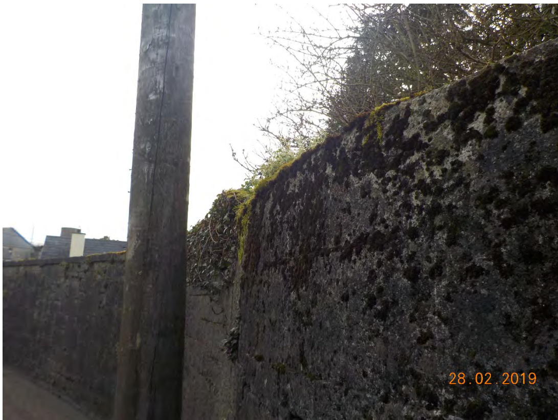
Photograph 3-8: Downstream Capping on Road Side Parapet
