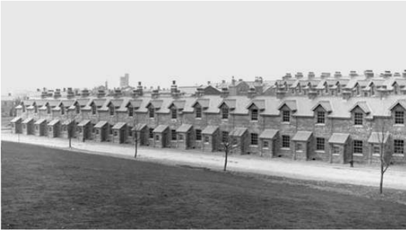
Figure 33 Married Quarters-Keane Barracks
