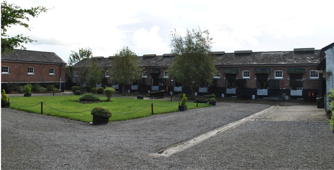
Survey 2_Figure 1 - Loose box stables viewed from general entrance
