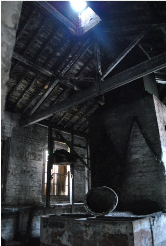
Survey 2_Figure 10 - View into Forge from Shed Showing original bellows mounted to rear
