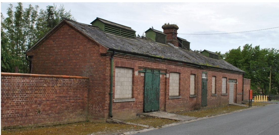
Survey 2_Figure 3 - Forge and Shoeing Sheds from Middle Road
