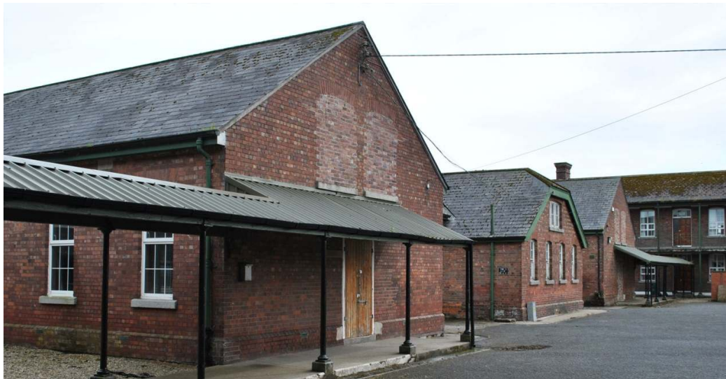
Survey 1_Figure 4 - Covered passage to dining hall and cookhouse
