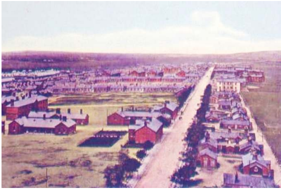
Figure 38 West side of camp from top of water tower after reconstruction.
