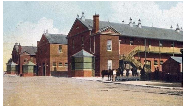
Figure 14 Cavalry accommodation blocks showing veranda access to first floor soldiers dorms, with stabling underneath.
