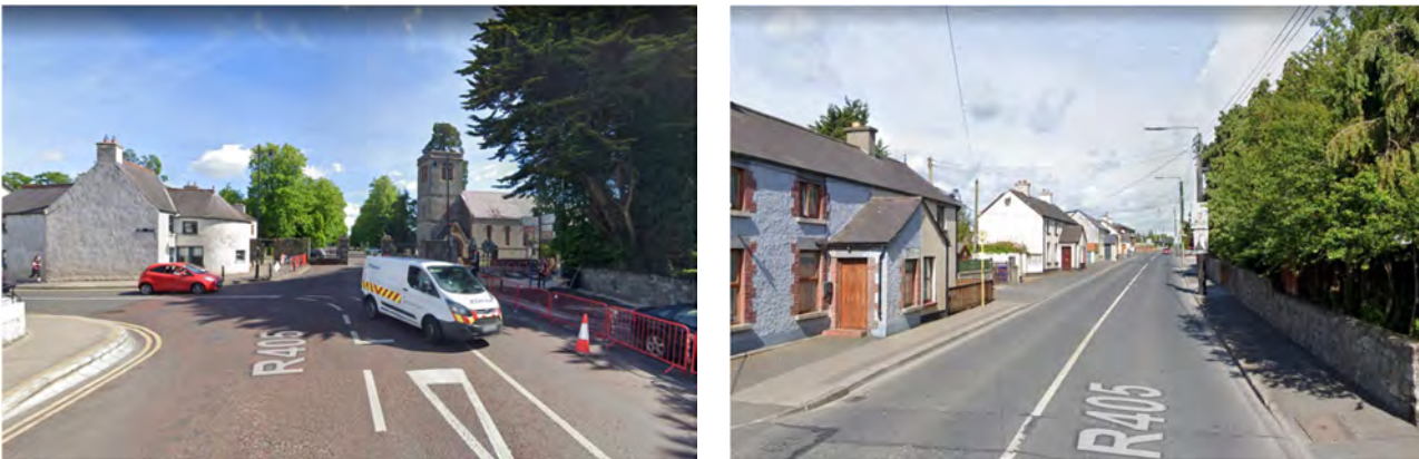
Figure 1-8: Main St & Maynooth Rd - Substandard Alignment and Cross Section and Concealed Property Accesses (Google Maps)
