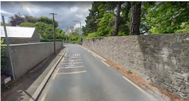
Figure 1-5: Newtown Rd & Existing River Liffey Bridge - Substandard Alignment and Cross Section (Google Maps)
