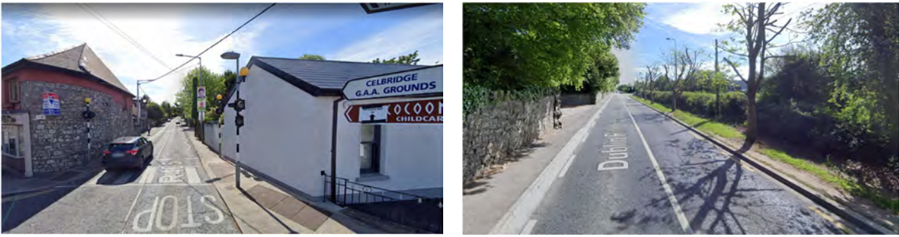
Figure 1-6: Hazelhatch Rd & Dublin Rd - Substandard Cross Section and Concealed Property Access (Google Maps)
