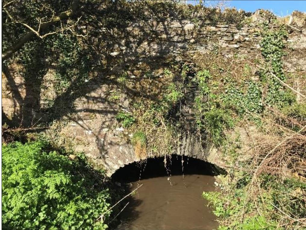
Figure 1: Moone Bridge Upstream Elevation
