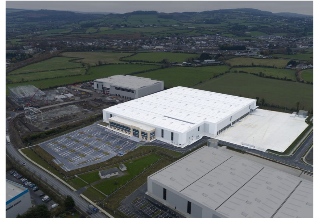
Building 2, Greenogue Logistics Park, Dublin
