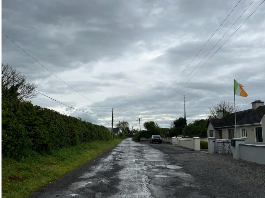
Fig. No.6 Road to west of the site which is a poor condition and has no footpath or lighting.
