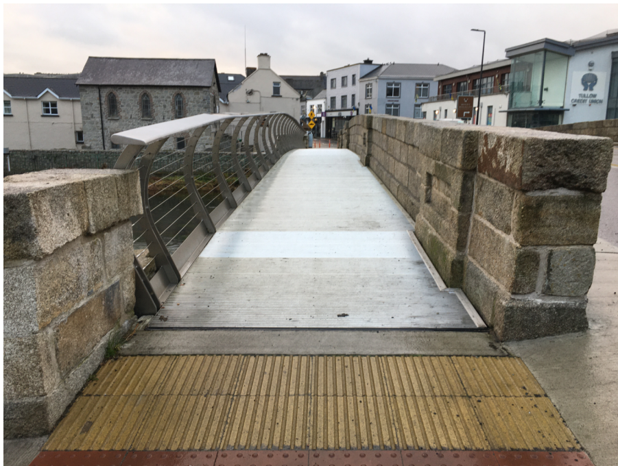
Figure 9: Image of the existing footbridge in Tullow over the River Slaney
