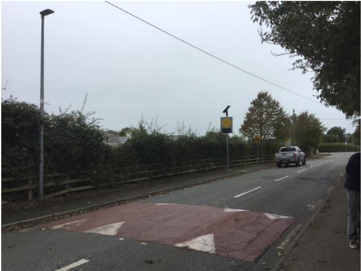
Figure 6. – As part of Planning permission granted works done to School Pedestrian Crossing
