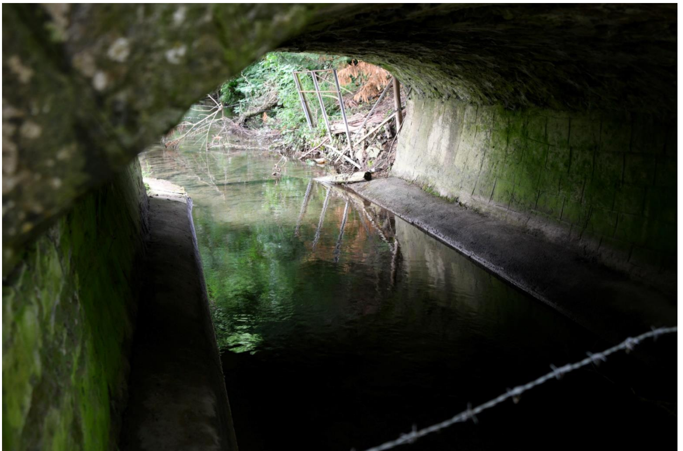
Plate 3. Mammal Passes under the bridge.
