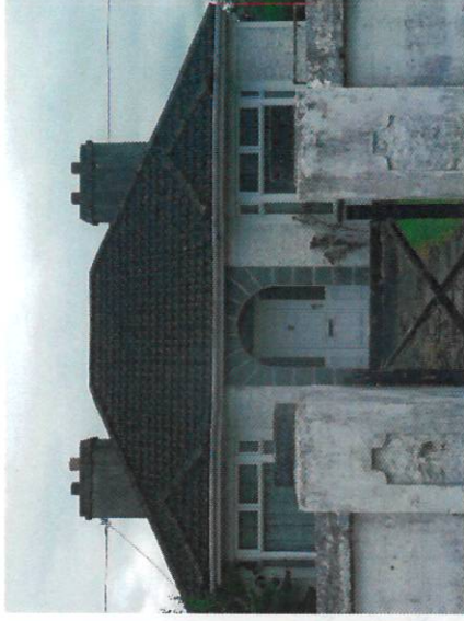
4.1. Note how the windows and door have changed in this detached three bay tiled hipped roofed bungalow from the 2003 NIAH survey
