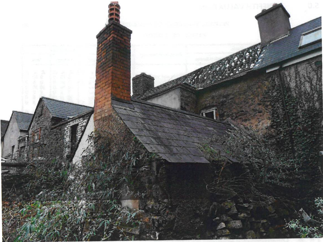
View of rear elevation of number 33 from rear garden of number 31
