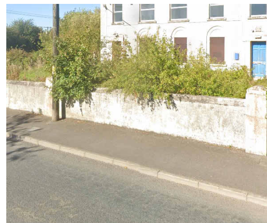
Mass concrete walls to front
