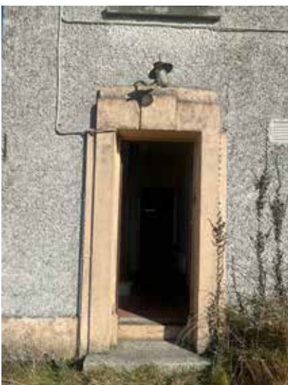
Fig.04 - External details - rendered doorset, cast rainwater goods, brick chimney
