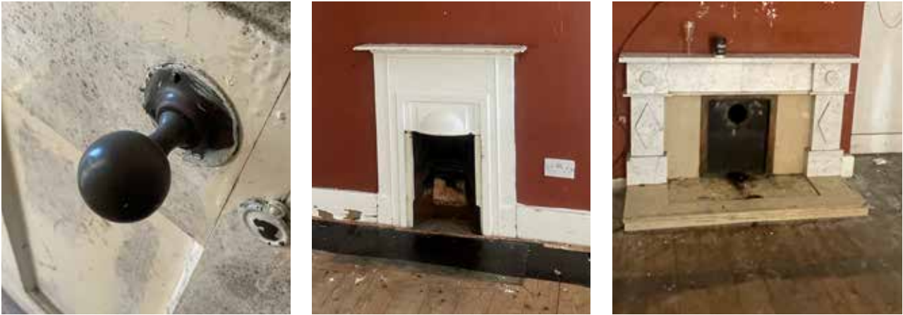
Fig.05 - Internal details including early doorsets and door furniture, fireplaces and surrounds
