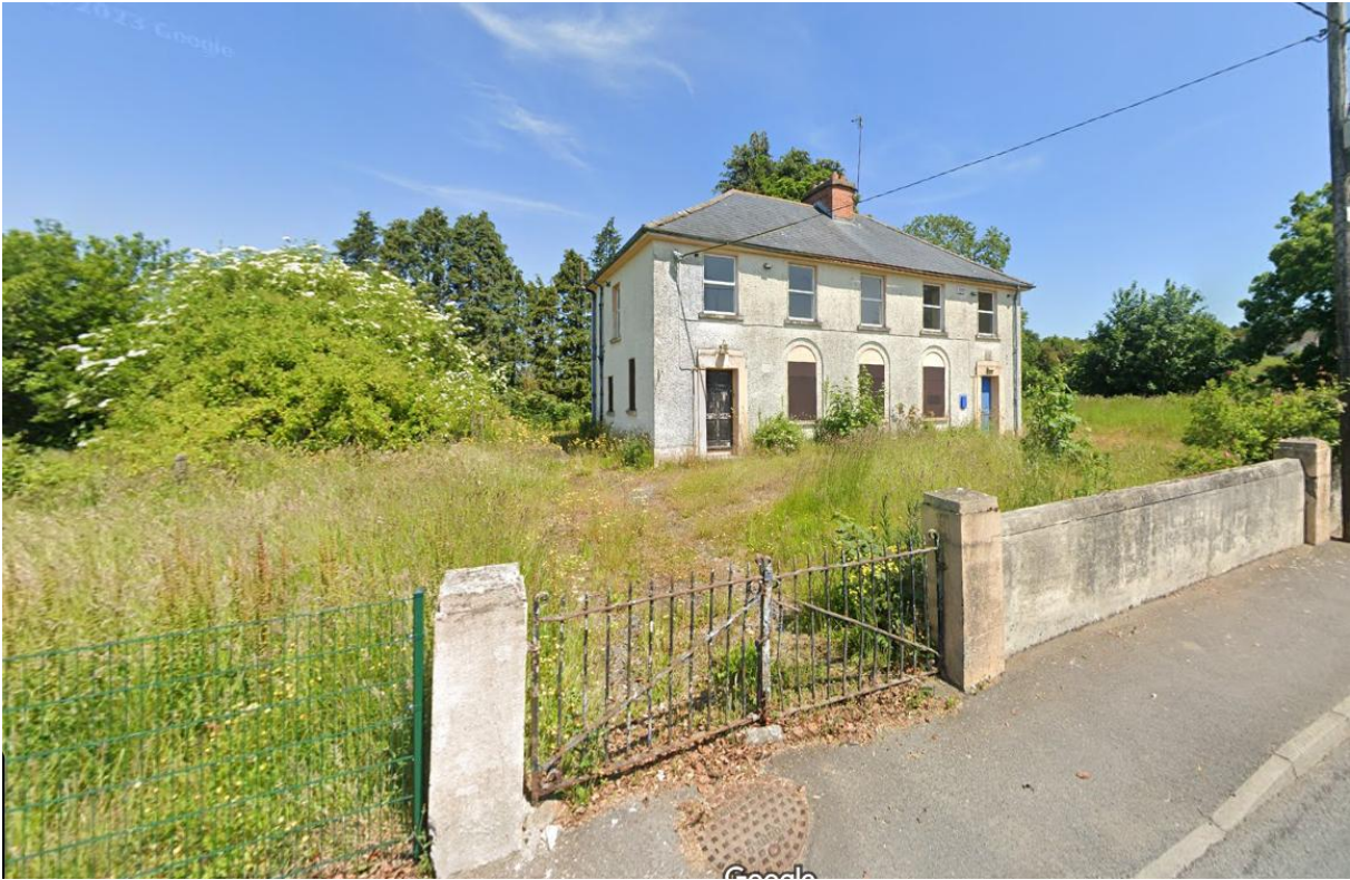
Figure 4: Recent condition of subject site – view from Barrack Road (Source: Google Street View)
