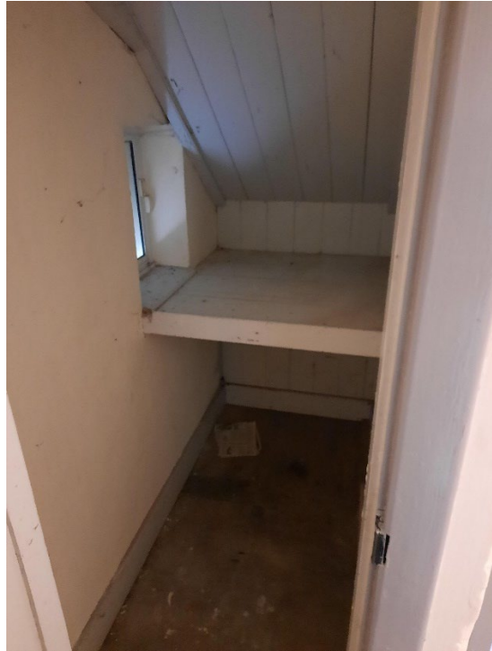
Photo G25 - Ground floor storage under stairs
