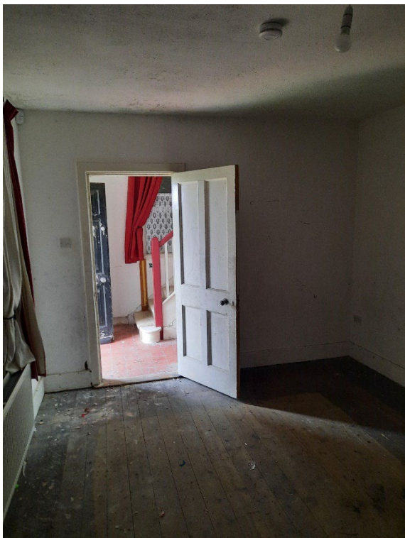
Photo G7 – Ground floor front room
