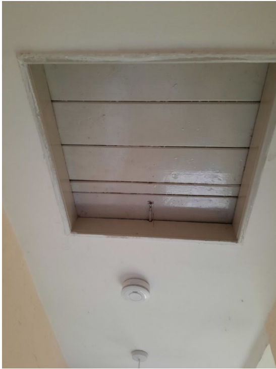
Photo G 30 First floor attic access
