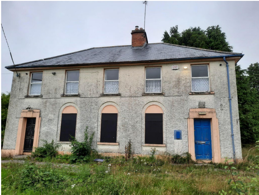
Photo G1 – Existing front elevation
