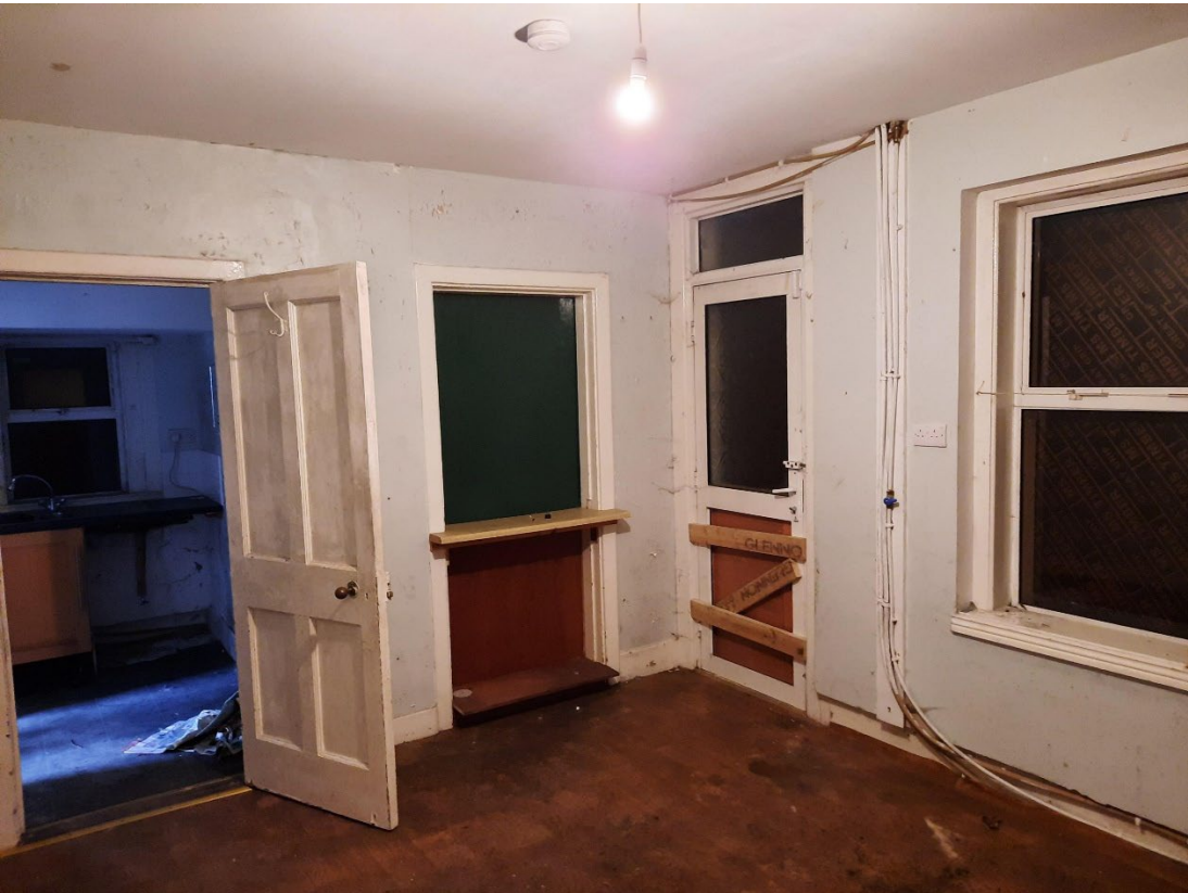
Photo G10 – Ground floor back room
