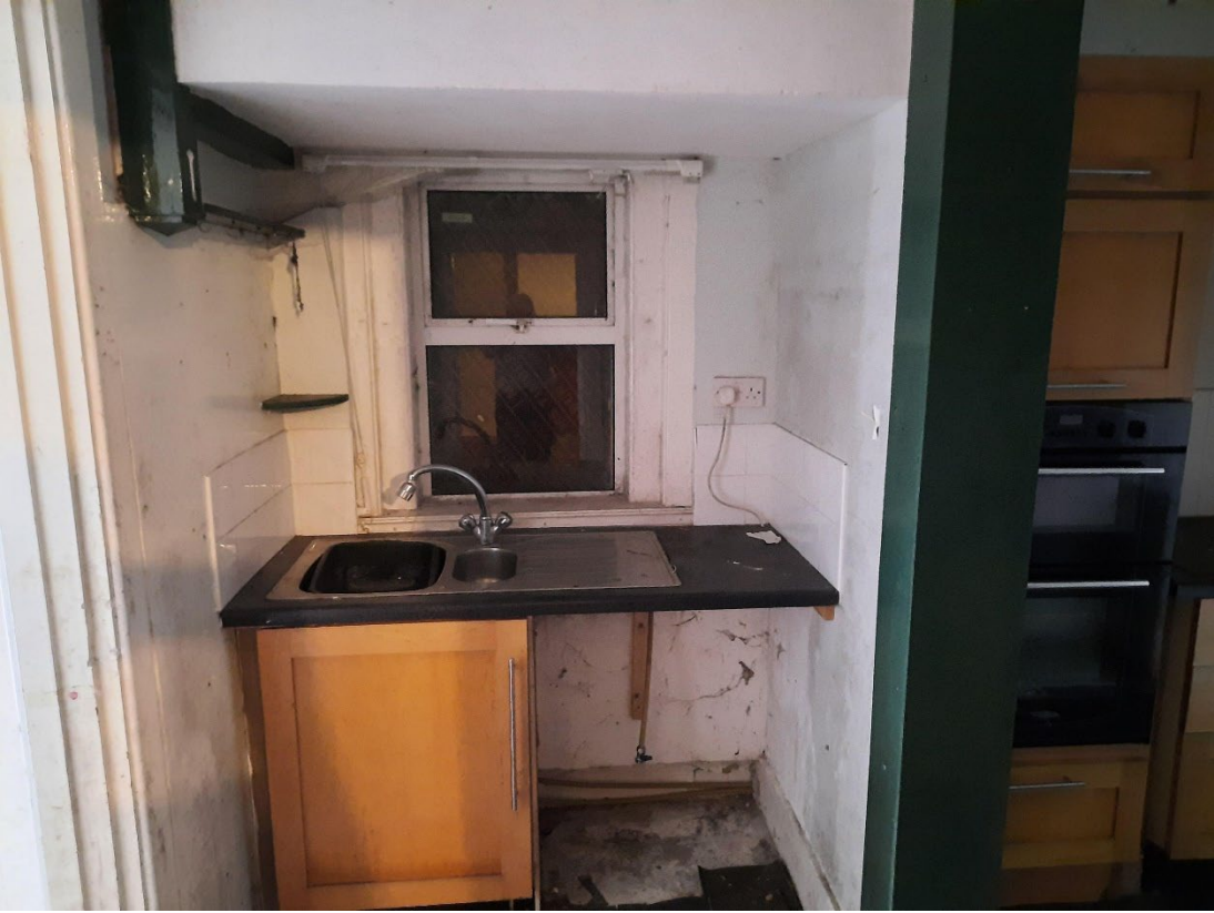
Photo G9 – Ground floor utility room
