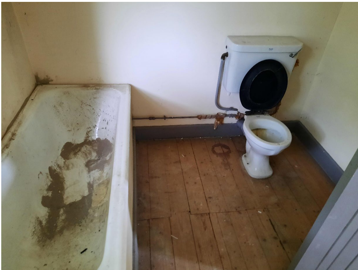
Photo G32 – First floor bathroom
