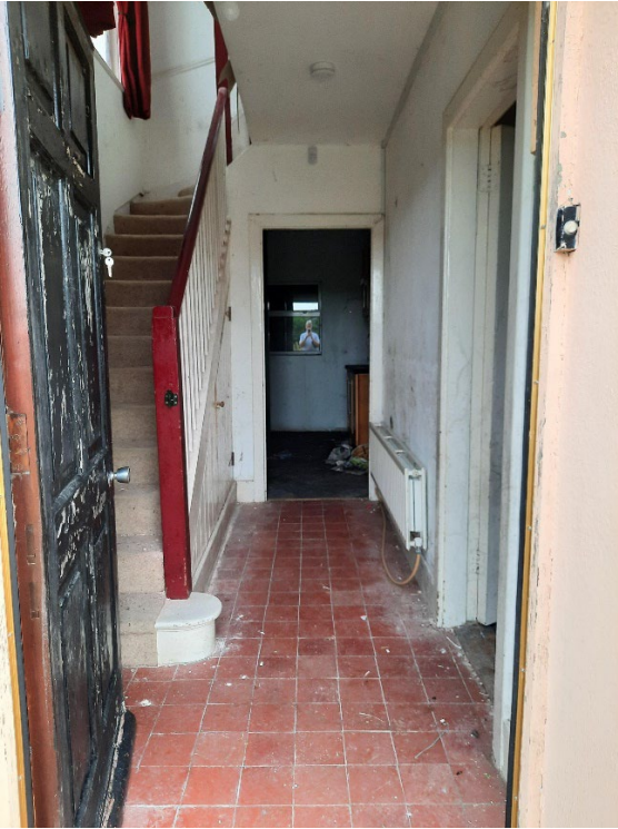
Photo G5 – Front entrance hall
