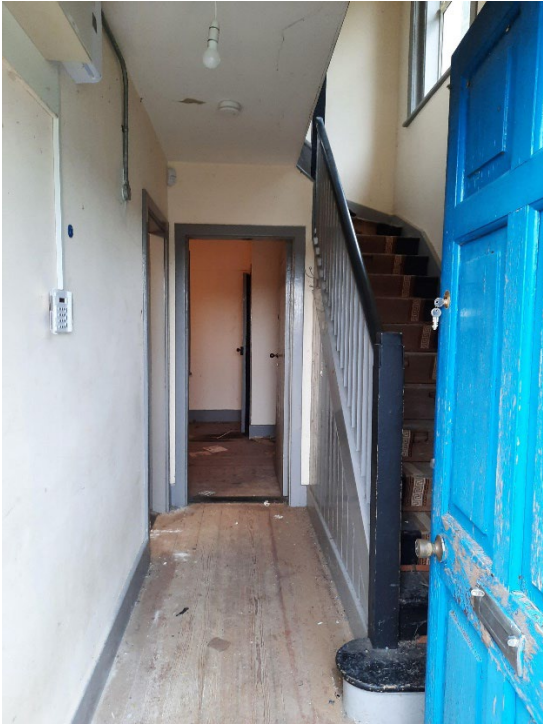
Photo G24 – Ground floor entrance hall
