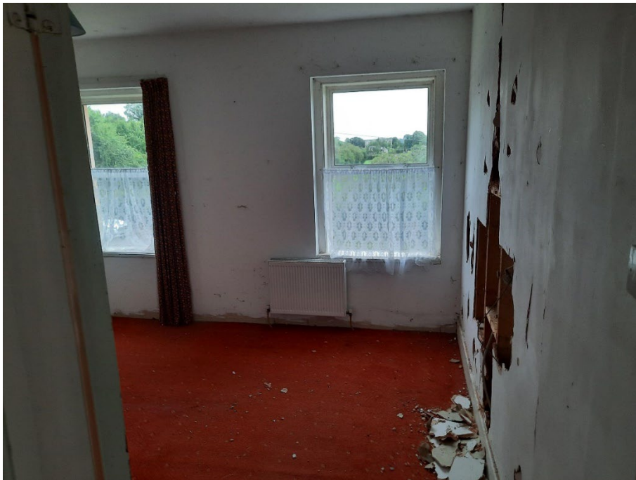
Photo G23 – First floor front bedroom
