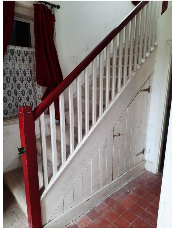
Photo G6 – Front entrance hall
