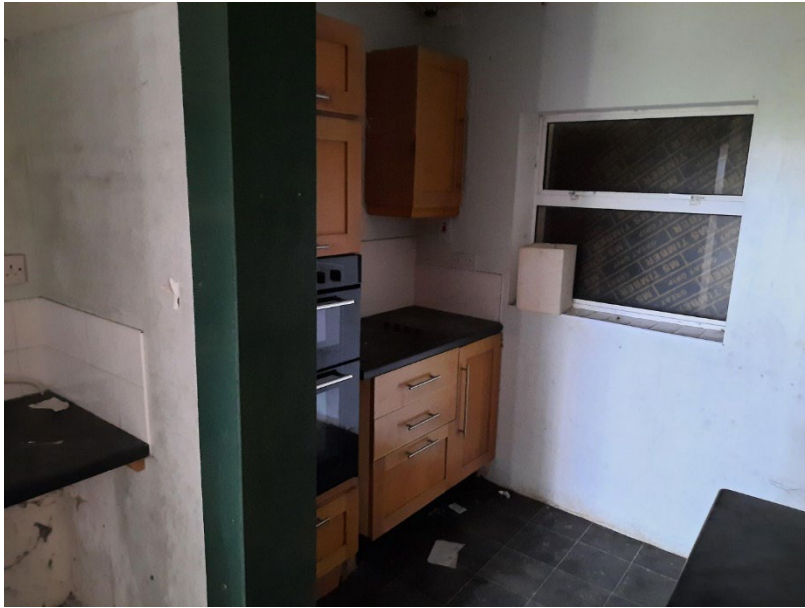
Photo G11 – Ground floor kitchen
