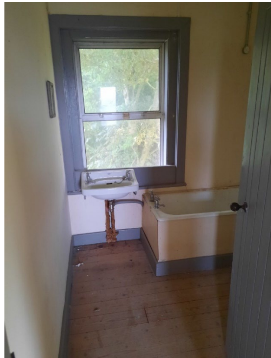
Photo G31 – First floor bathroom
