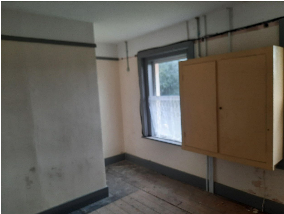
Photo G34 – First floor back office
