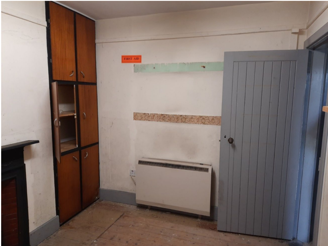
Photo G26 – Ground floor front office
