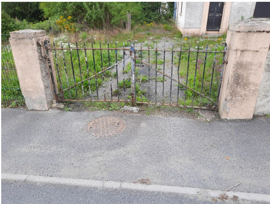
Photo G2 – Existing site access
