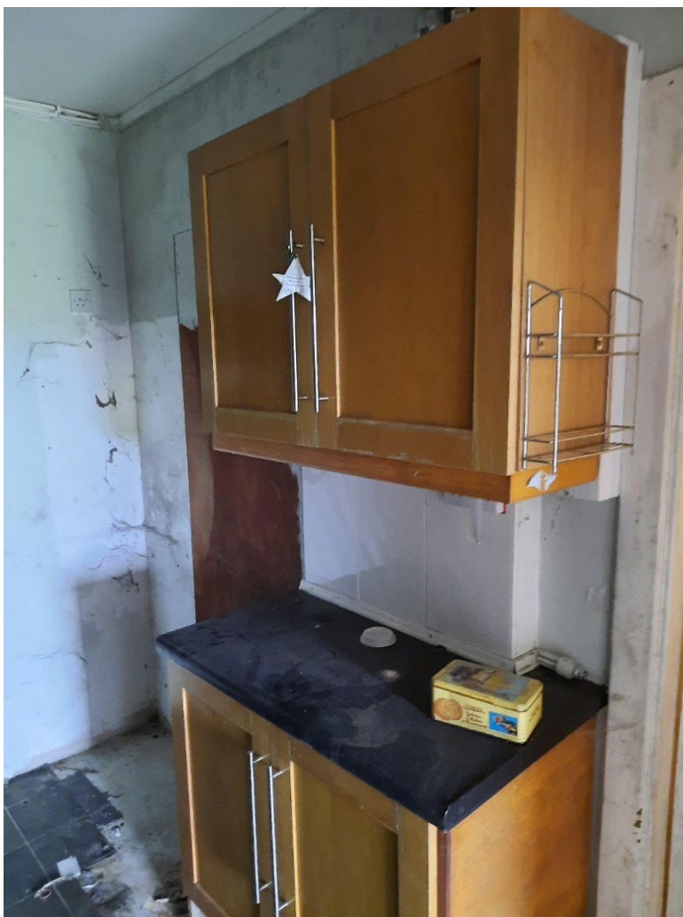
Photo G12 – Ground floor kitchen
