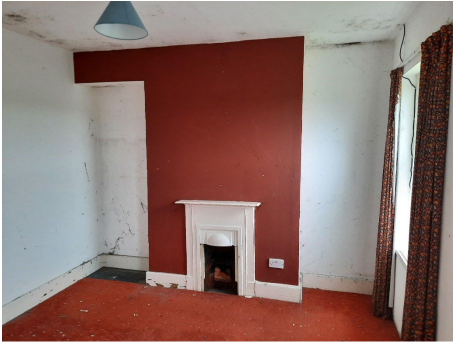
Photo G22 – First floor front bedroom
