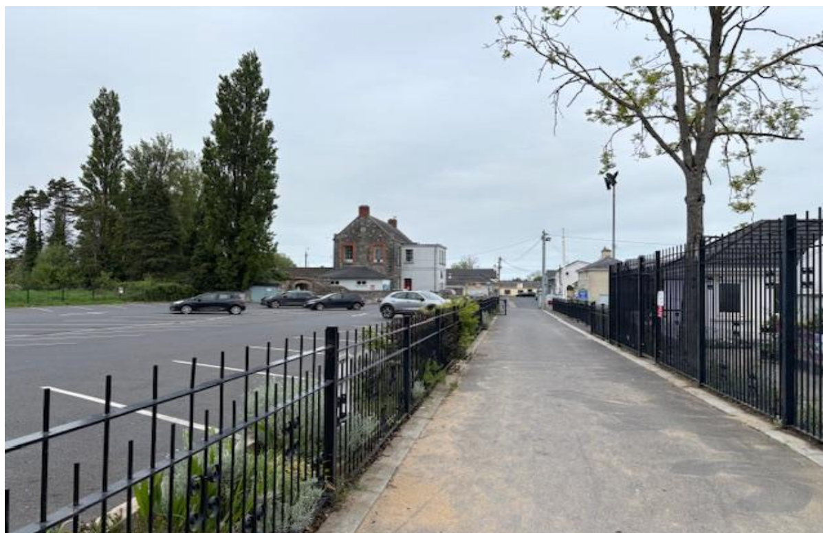
Figure 9: Sallins Community Centre/Parish Hall
