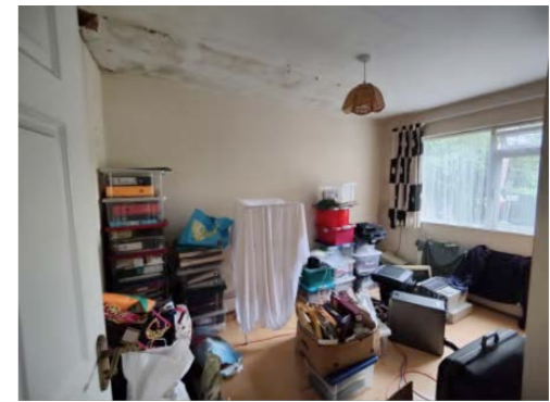
2001_Beaufort Cottage_Room 124_IMG20240712111852.jpg
