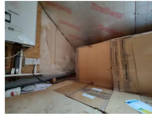
2001_No 18_Room 162 Attic_IMG20240712113349.jpg
