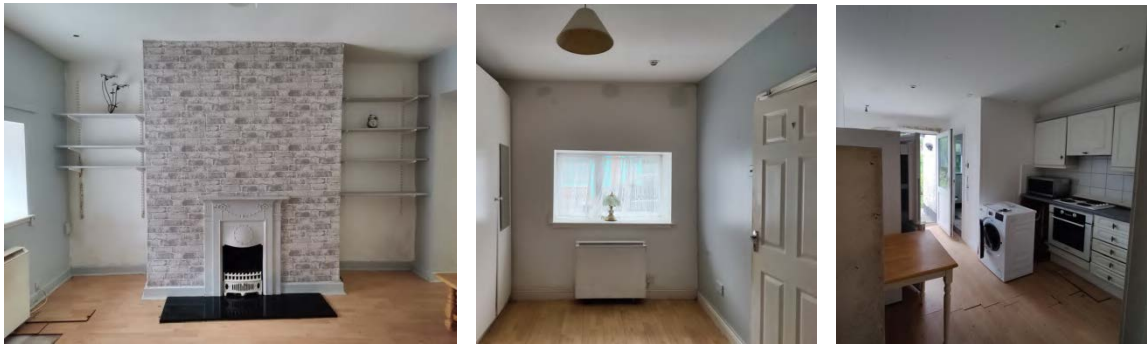
Above: Photographs showing the interior of 13 Sallins Road taken in July 2024. All wall, floor and ceiling finishes are modern replacements.
