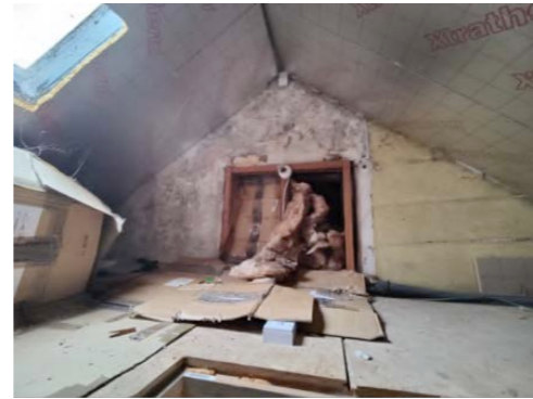
2001_No 18_Room 162 Attic_IMG20240712113342.jpg
