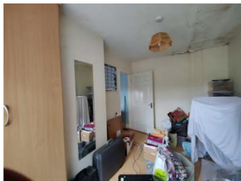
2001_Beaufort Cottage_Room 124_IMG20240712111905.jpg
