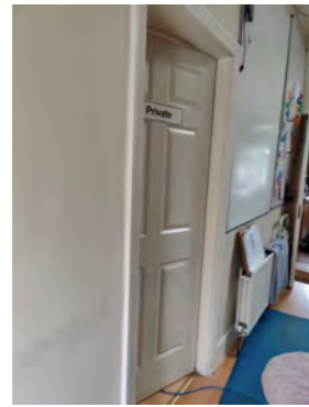
2001_Beaufort Cottage_Room 121_IMG20240712111736.jpg
