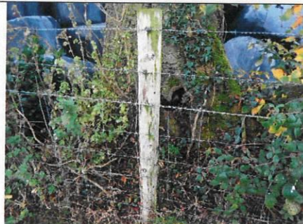
Cavity at base of Ash tree T22
