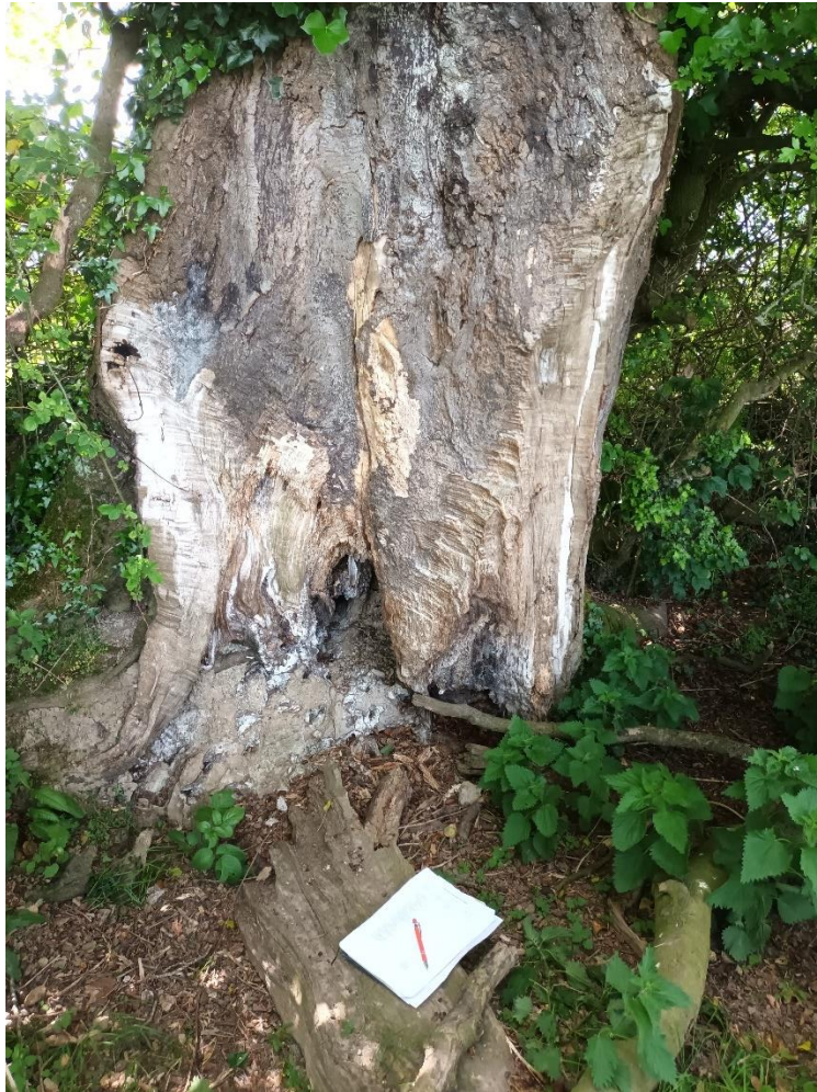
Significant Damage at the buttress of 0610
