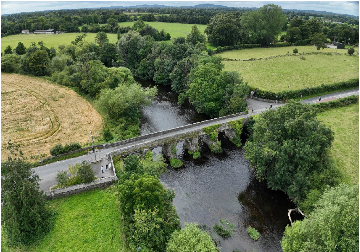
PHOTO 2-7 AERIAL IMAGE OF CARAGH BRIDGE (KILDARE COUNTY COUNCIL)
