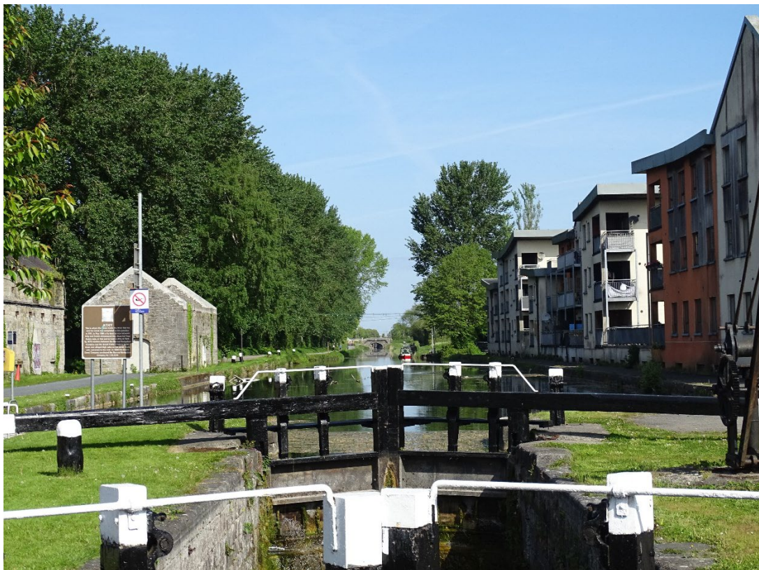
PHOTO 2-13 VIEW NORTHWARDS ALONG THE GRAND CANAL – BARROW LINE, ATHY
