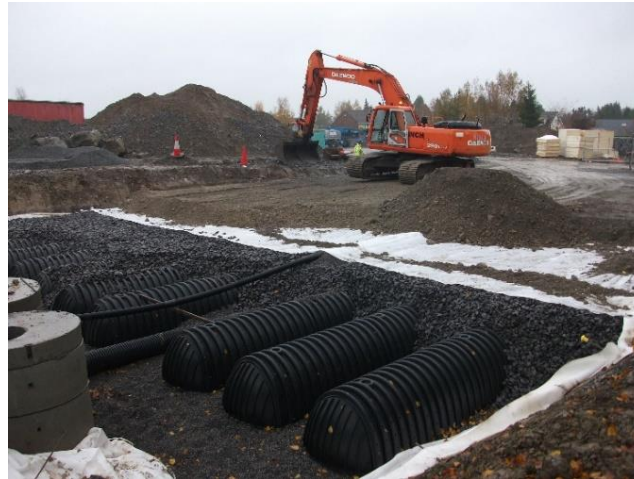
Figure 9-2: Typical attenuation/soakaway structure
