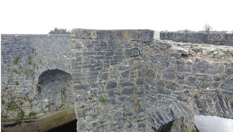
PHOTO 03 UPSTREAM SPAN 1 DAMAGED CUTWATER/CRACKING
