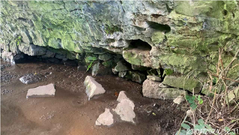
PHOTO 04 RELIEF ARCH UNDERMINING / COLLAPSED ABUTMENT
