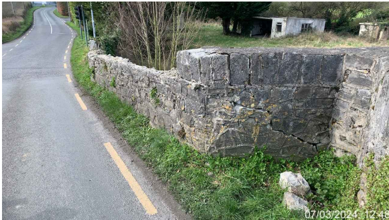
PHOTO 02 UPSTREAM SPAN 1 DAMAGED PARAPET
