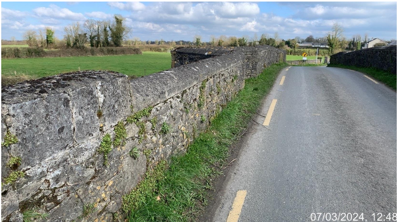
Figure 8 Minor Vegetation Growth and Missing Pointing, Parapets, looking north
