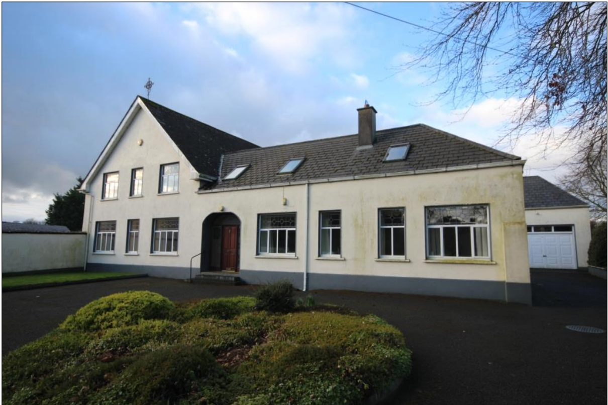
Plate 3: View of the front elevation of the former convent
