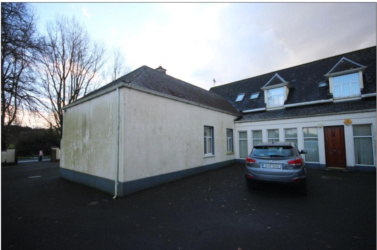
Plate 4: View of the rear elevation of the original single-storey element of the former convent. The dormer extension to the rear (on the left of the photograph) is a later twentieth-century addition.
