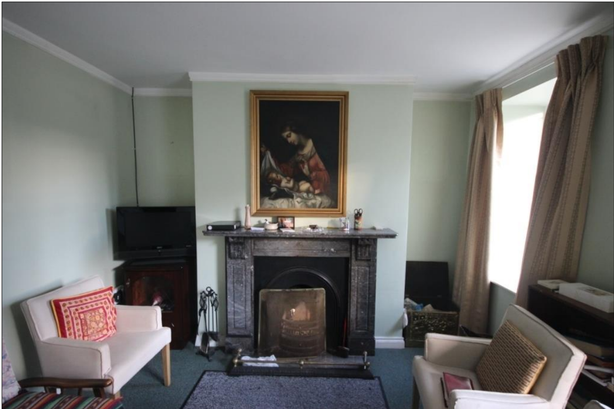
Plate 9: Living room to the east of the entrance hall. The ceilings, wall surfaces and floor have been modernised. The fireplace is late insertion.
