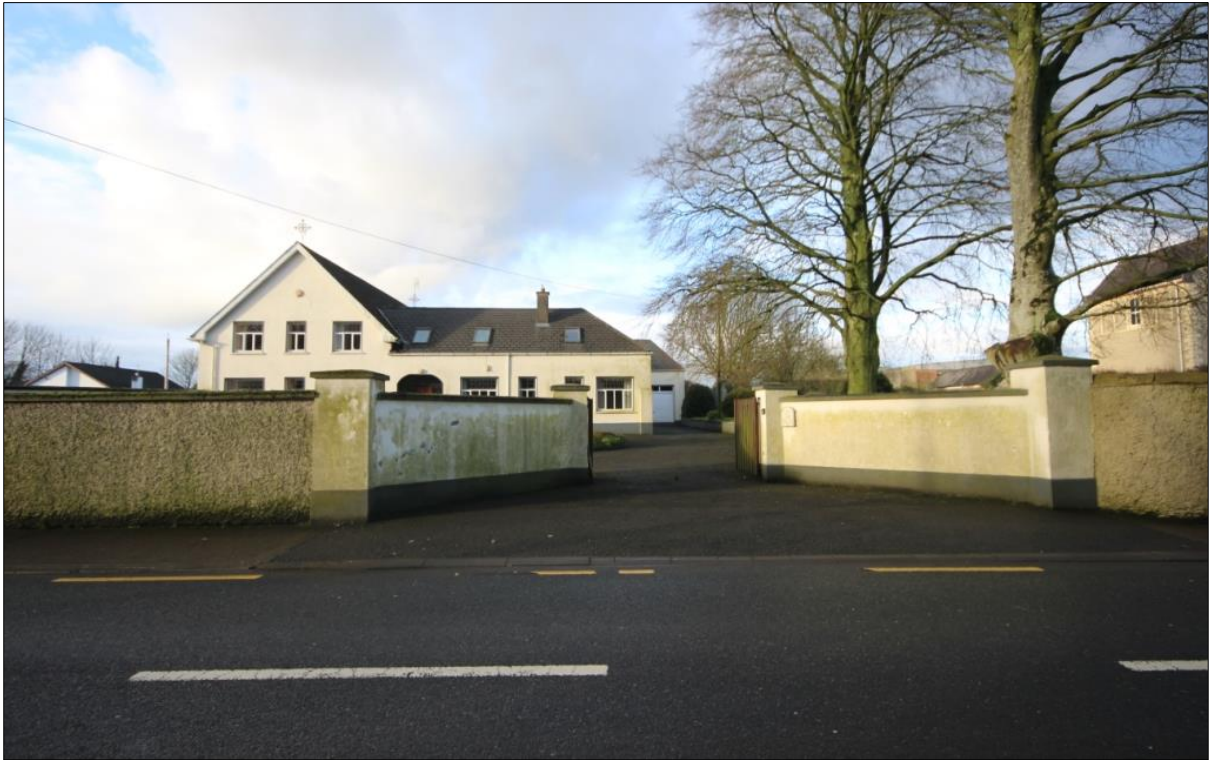
Plate 1: View of the entrance way to the former convent
