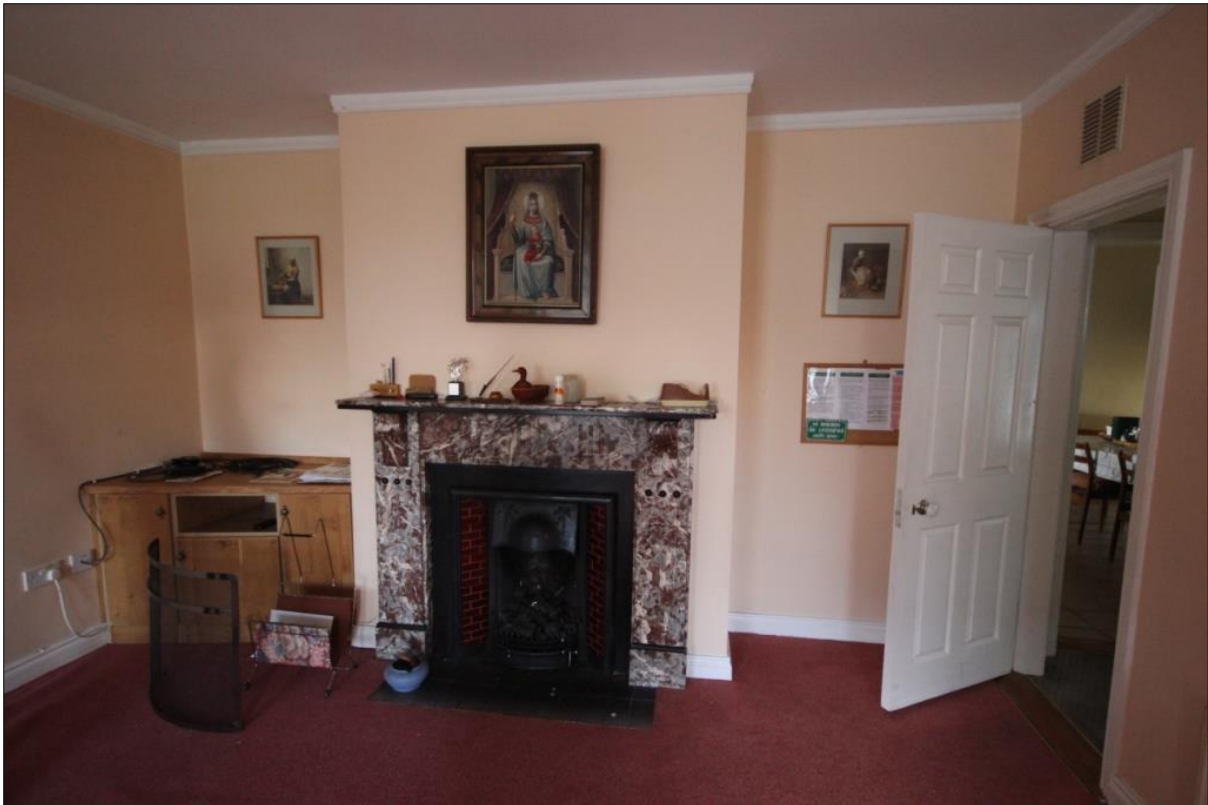
Plate 11: Living room to the west of the entrance hall. The ceilings, wall surfaces and floor have been modernised. The fireplace is late insertion.
