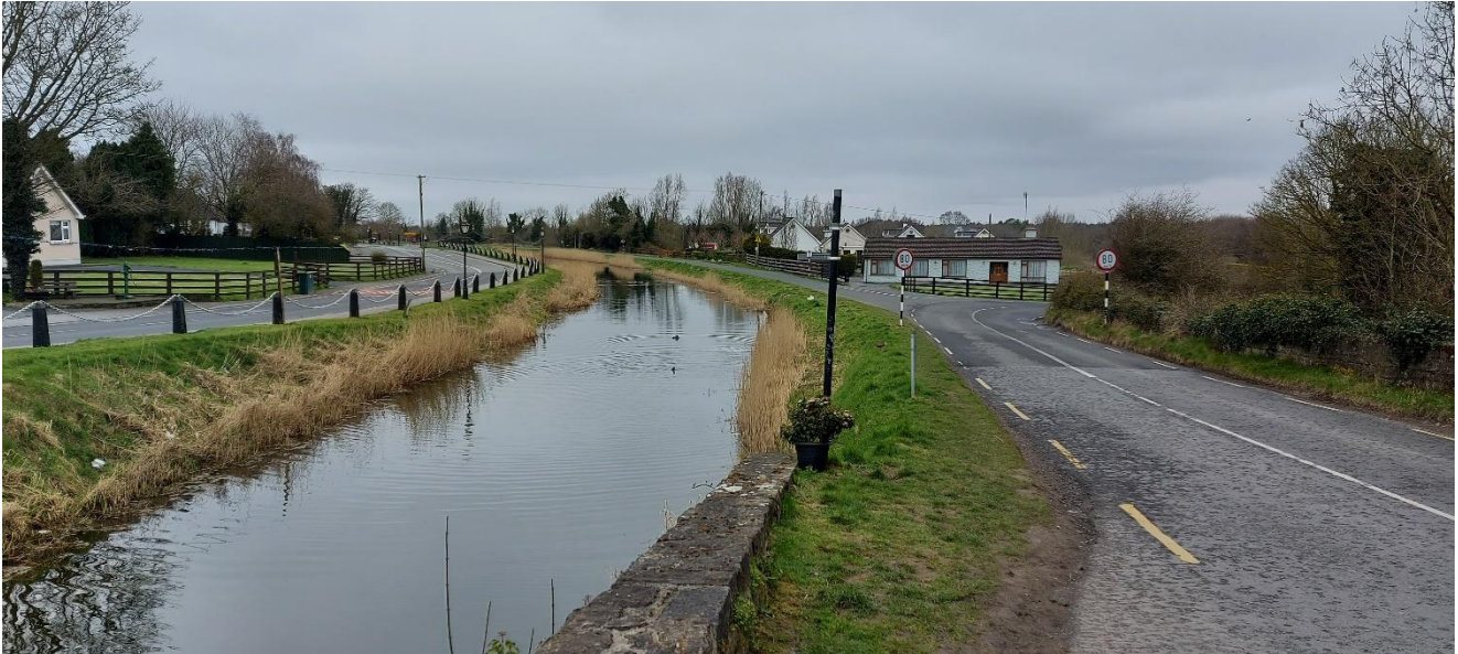
Figure 3-2: View along the L7073 facing west (note the sharp right hand bend where the greenway user would have to turn off onto the L7073-5)
