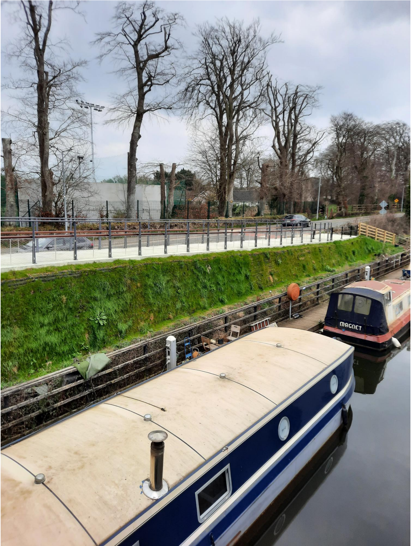
Figure 3-8: Green Faced Reinforced Earth Approach Ramps (Sallins)
