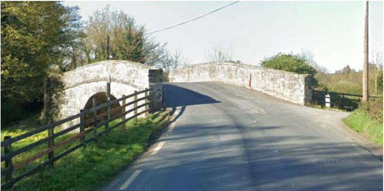
Figure 3-5: Bonynge/Healy's Bridge View from South (note lack of appropriate sightlines)
