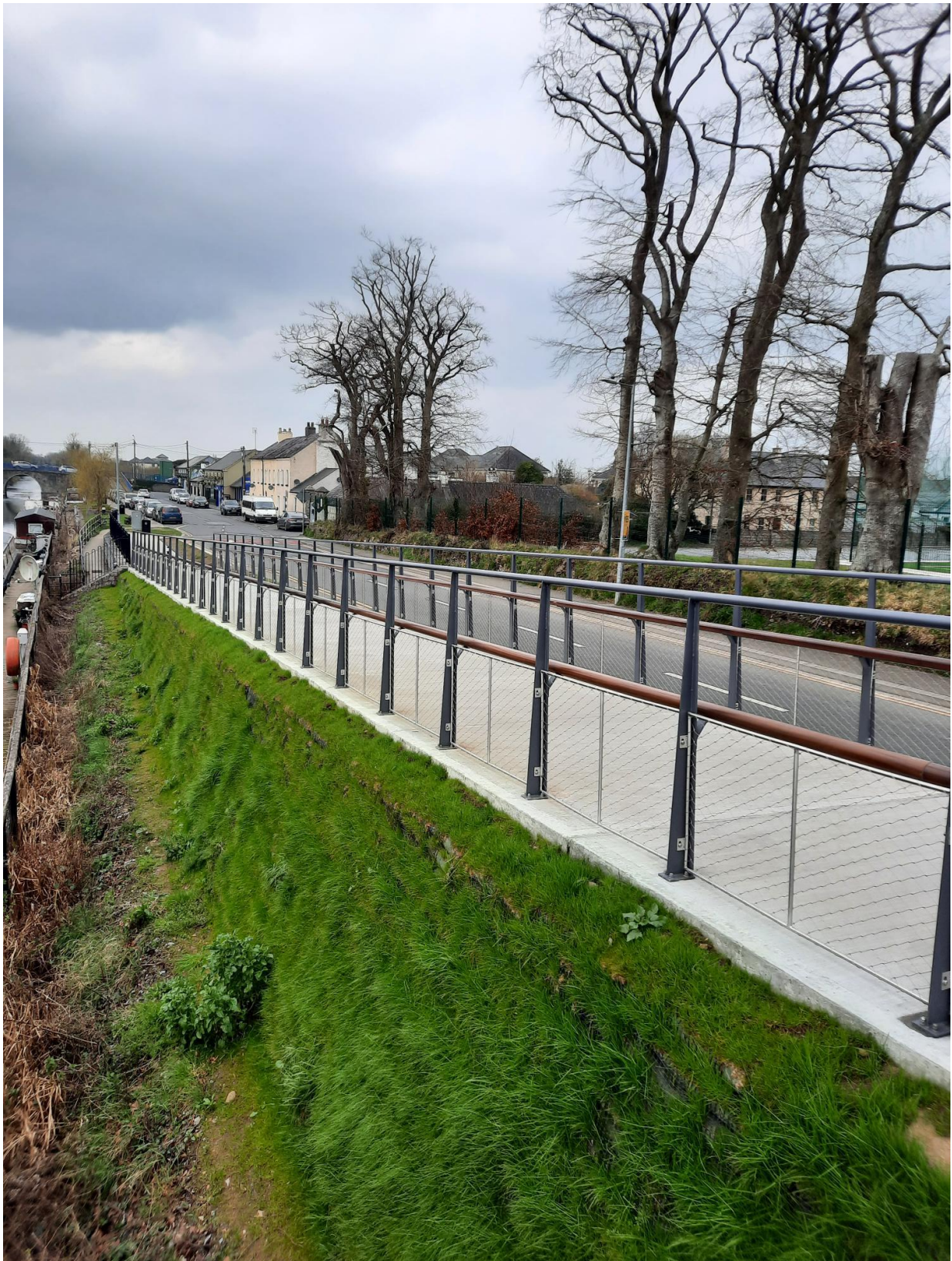
Figure 3-9: Grassed Finish to Pedestrian Approach Ramps at Sallins Bridge
