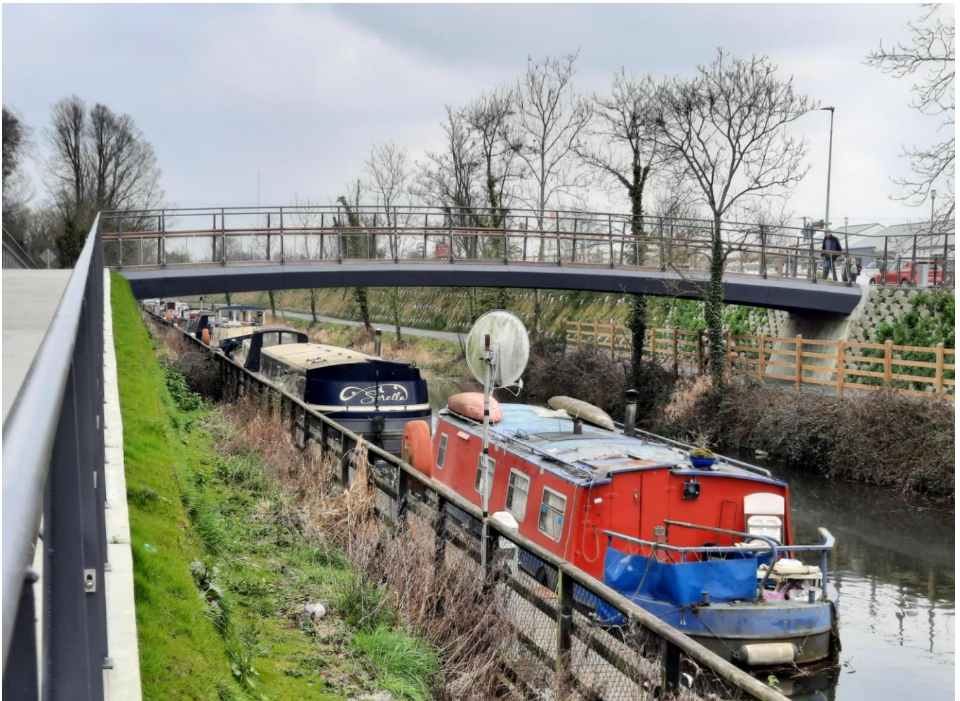
Figure 3-7: Simple Curved Steel Bridge Recently Installed at Sallins
