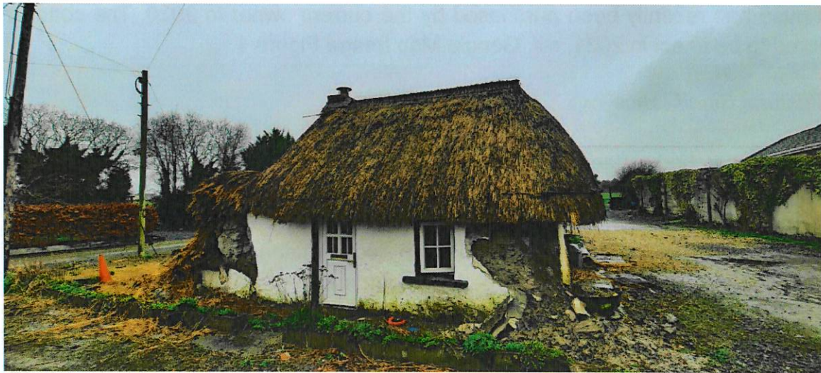
Figure 2: Current condition of thatched cottage facing south
