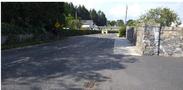
View of Ardclough Rd. north of Pausdeen Bridge, looking towards Celbridge (to the North)
