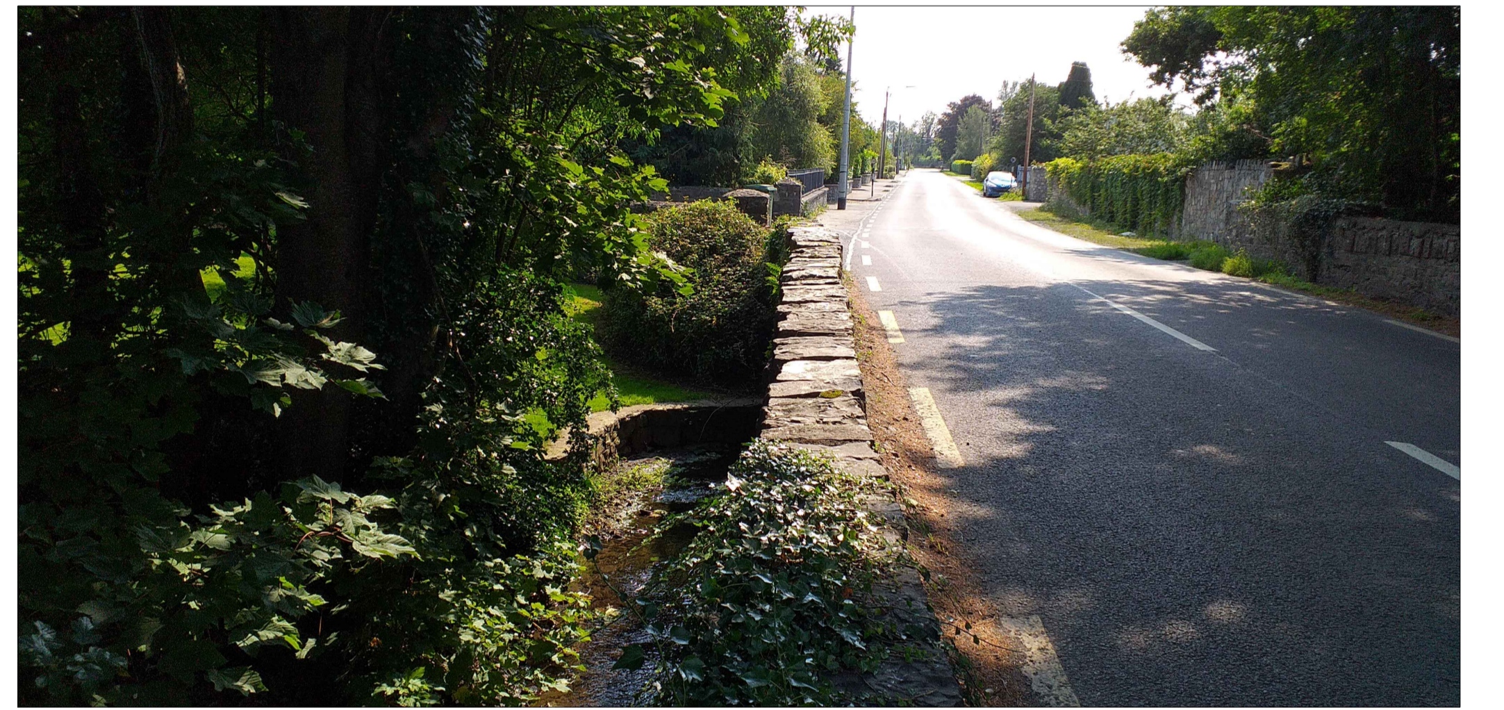
Existing Pausdeen Bridge (View from North to South)
