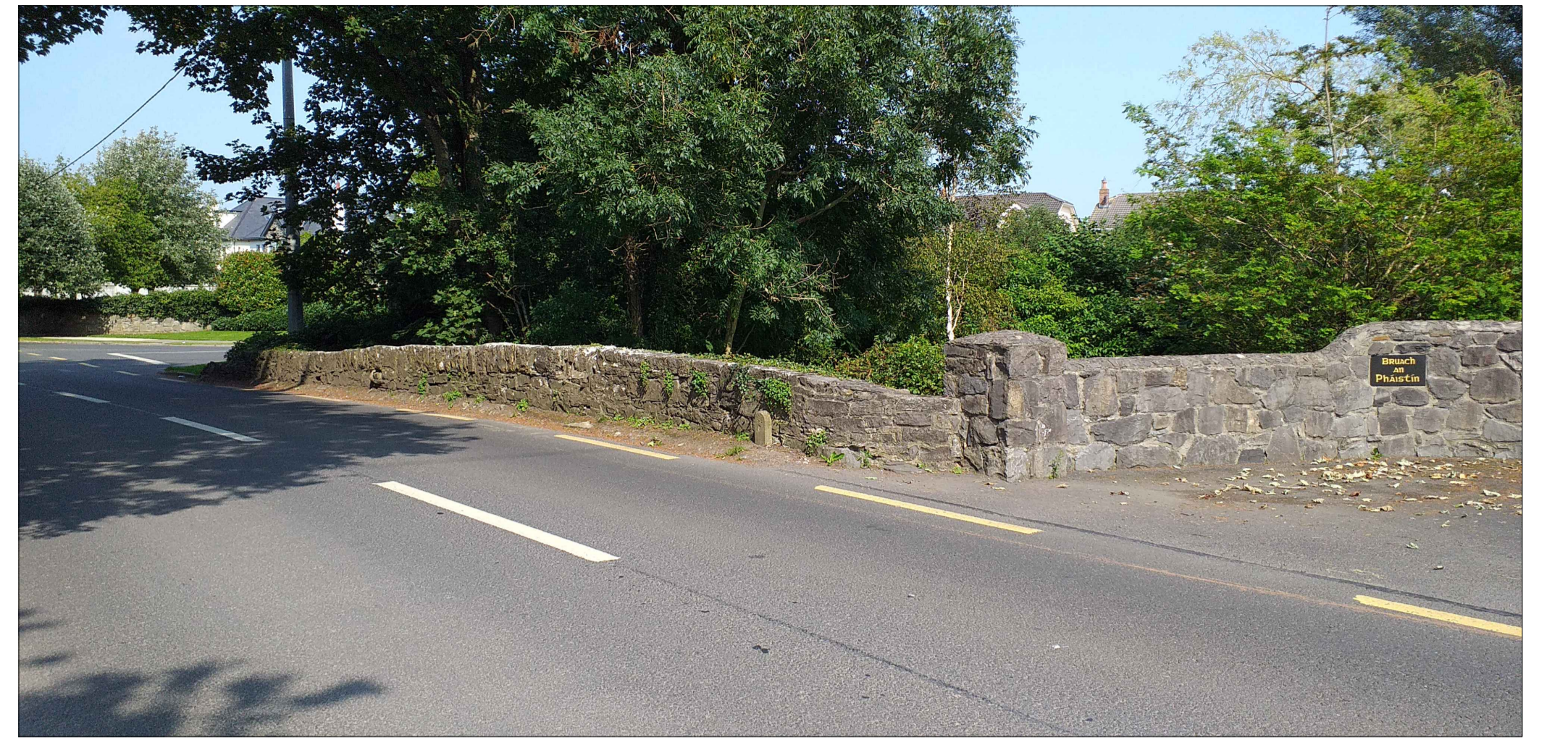
Existing Pausdeen Bridge (View from Southeast to North East)
