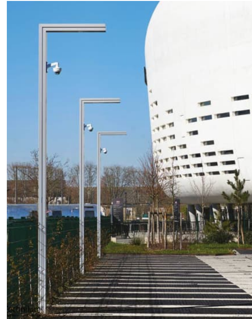
Figure 3: Main Street Lighting TECHNILUM SHIRAZ (K)
