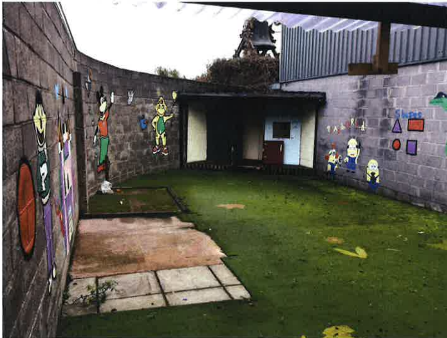
Figure 2 View from the garden, Unit 8&9, The Village Centre, Clane
