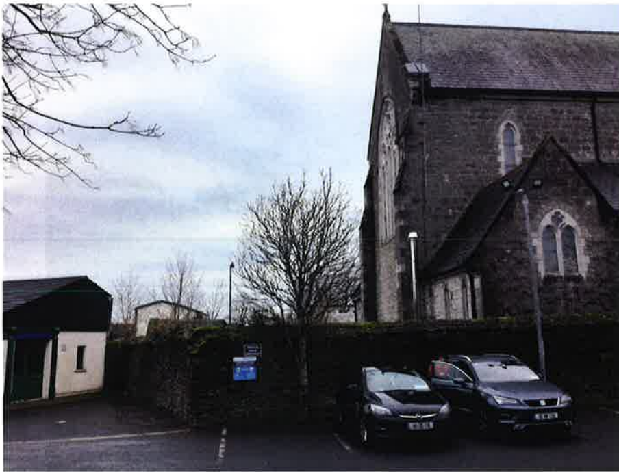
Figure 3 View from the end of the car park, The Village Centre, Clane
